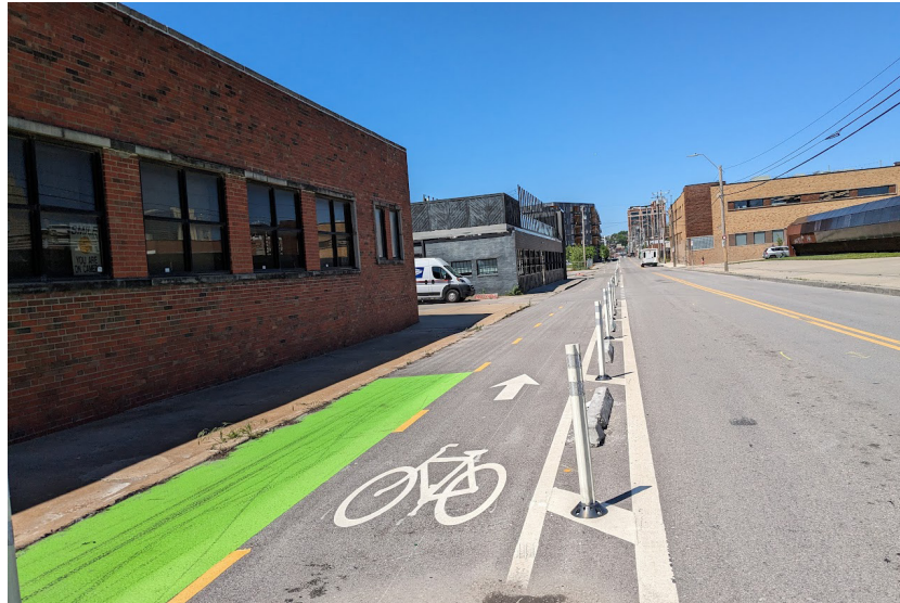
Figure 3 – Two-way cycle track using quick-build materials
