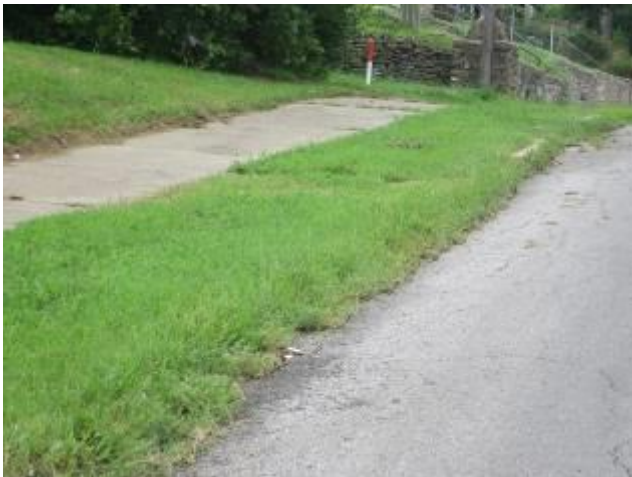
Lack Of Curbs &amp; Gutters Along College Avenue
