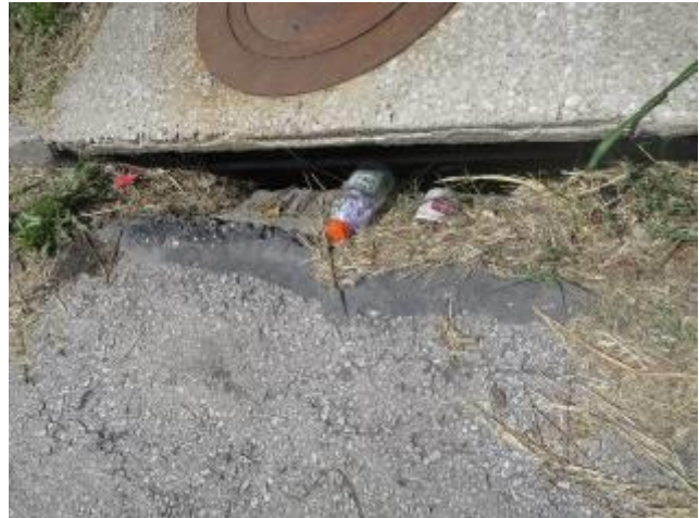
Clogged Sewer Inlet Along E 49 th Street
