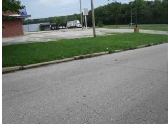
Deteriorating Curbs Along College Avenue
