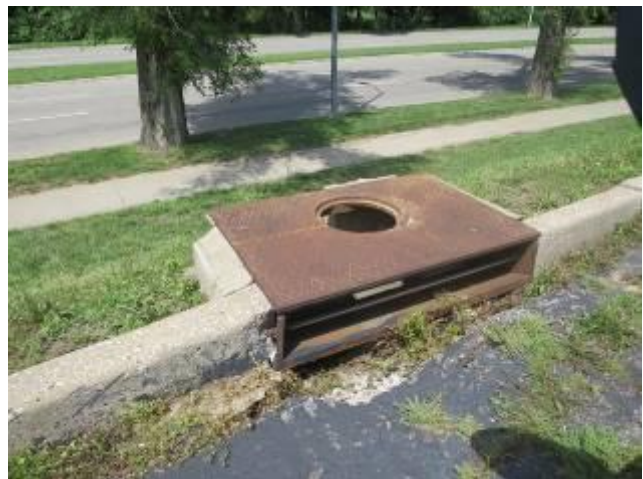
Deteriorating Sewer Inlet At 3011 Swope Parkway
