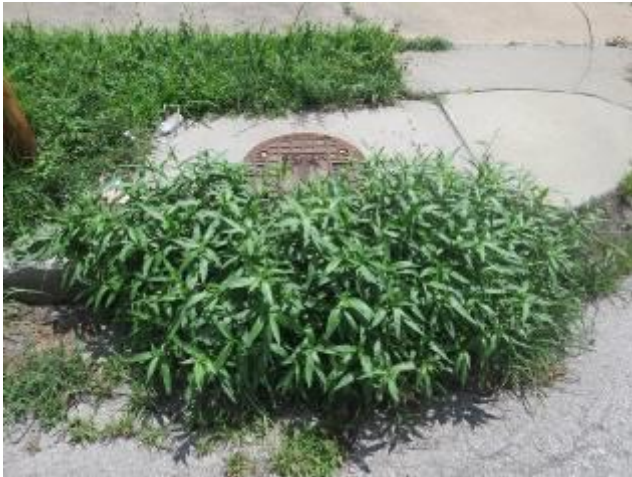
Clogged Sewer Inlet Along E 49 th Street
