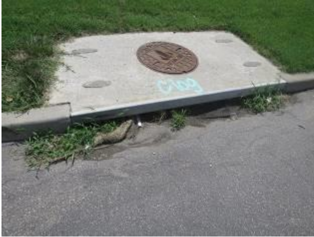
Clogged Sewer Inlet Along Swope Parkway
