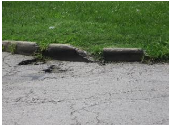
Deteriorated Curbs Along Agnes Avenue
