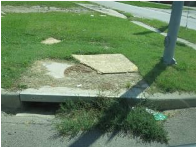
Clogged Sewer Inlet Along Swope Parkway
