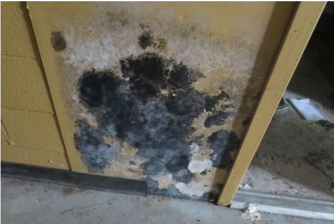
Water Infiltration And Black Mold – 2801 Swope Parkway
