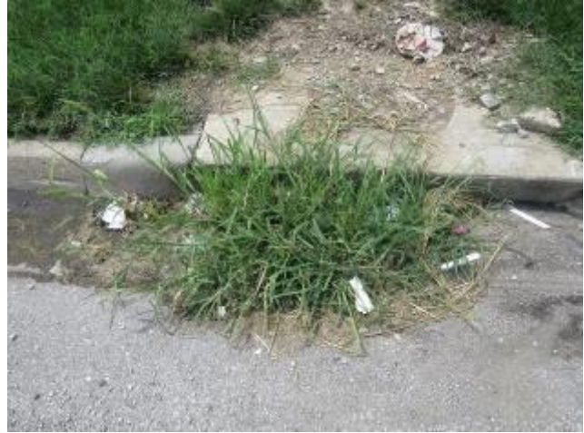
Clogged Sewer Inlet Along Chestnut Avenue
