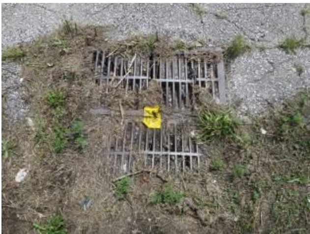
Clogged Sewer Inlet At 2801 Swope Parkway
