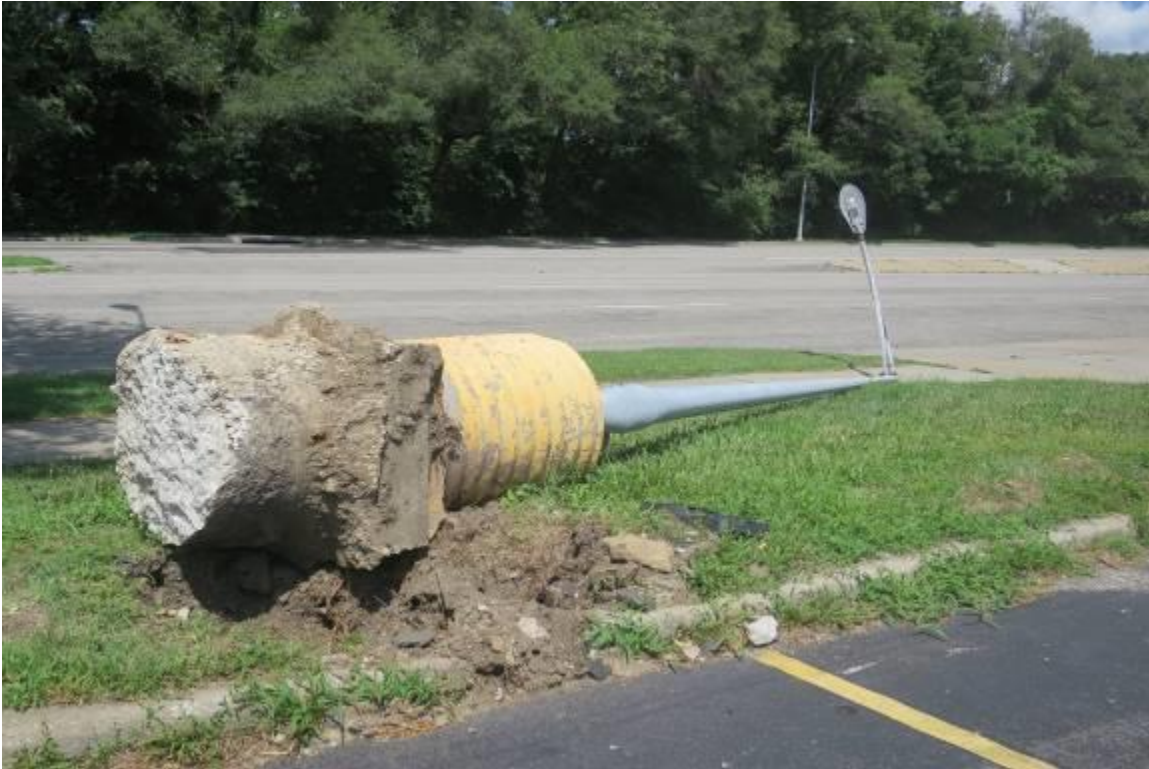
Collapsed Parking Lot Lamppost – 3011 Swope Parkway
