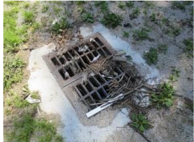
Clogged Sewer Inlet At 3011 Swope Parkway
