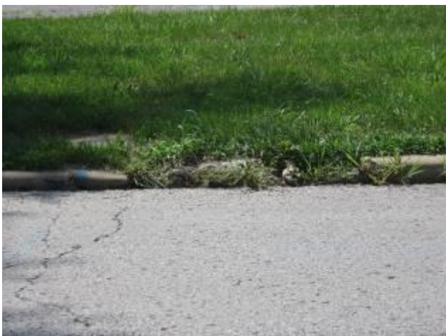
Deteriorated Curbs Along Agnes Avenue
