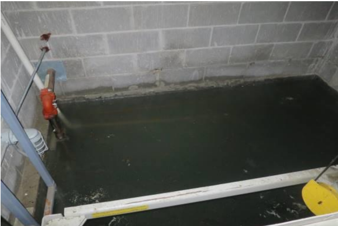
Water-Filled Elevator Shaft – 2801 Swope Parkway
