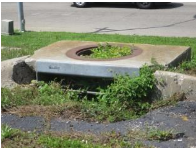
Clogged Sewer Inlet At 3011 Swope Parkway
