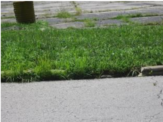
Deteriorated Curbs Along Agnes Avenue
