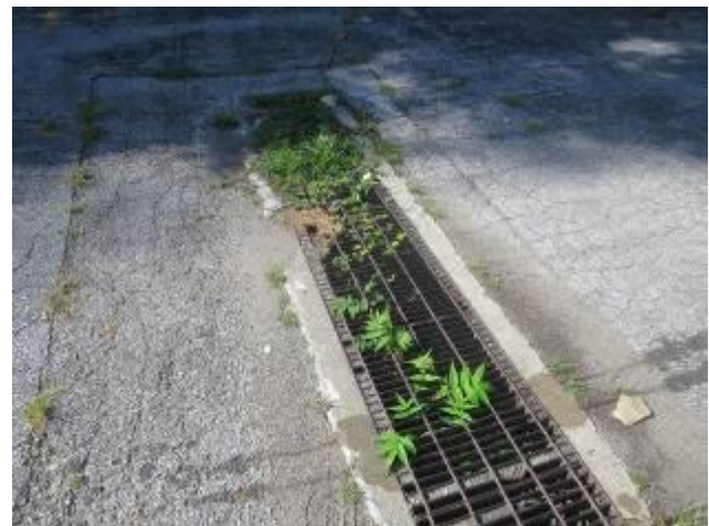
Clogged Drainage Grate At 2915 Swope Parkway
