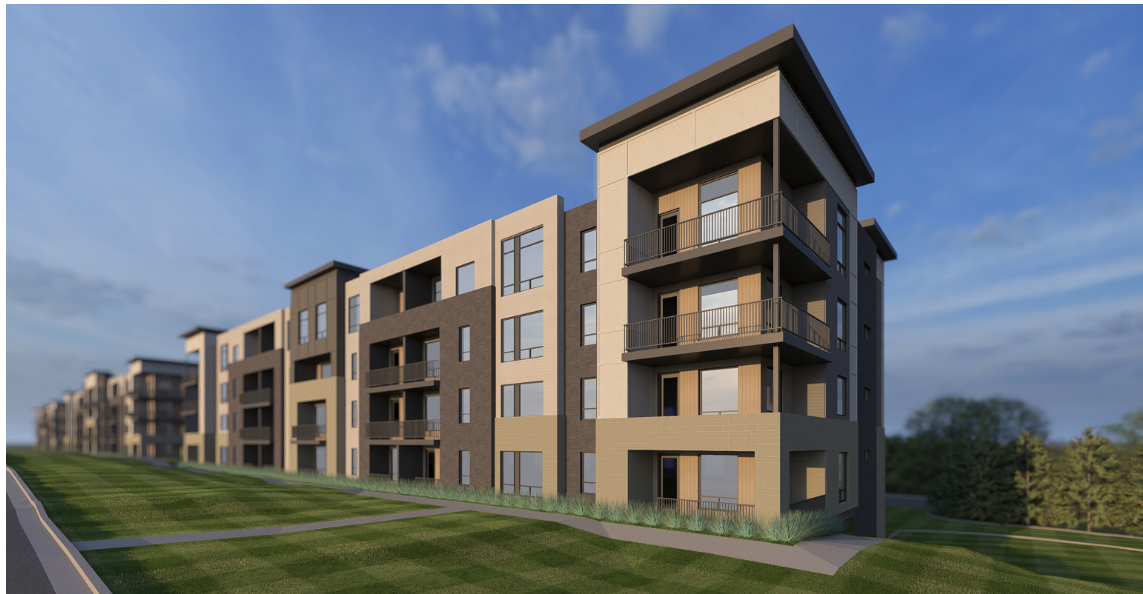
VIEW 1 - SOUTH END BUILDING 1
