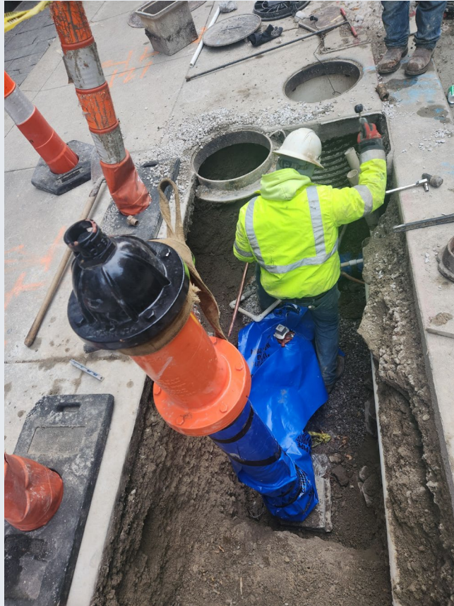
Emergency Distribution Repairs
