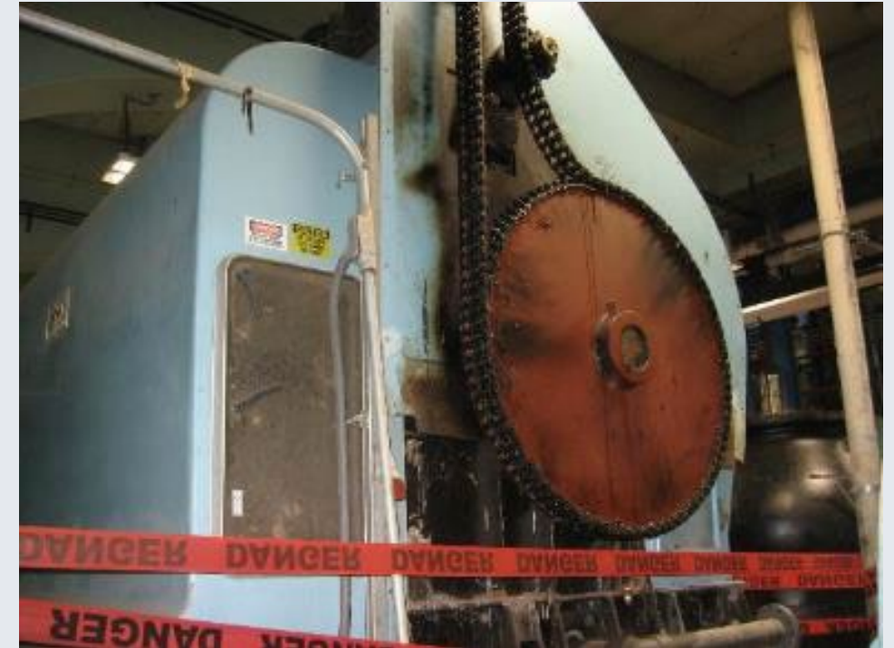
Housing for the River Intake Traveling Screens
