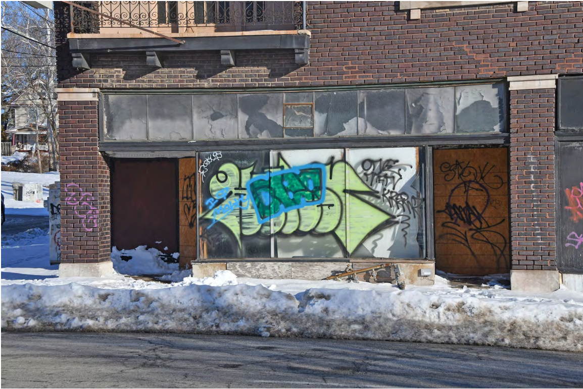
03: Exterior, west elevation, north storefront, view E.
