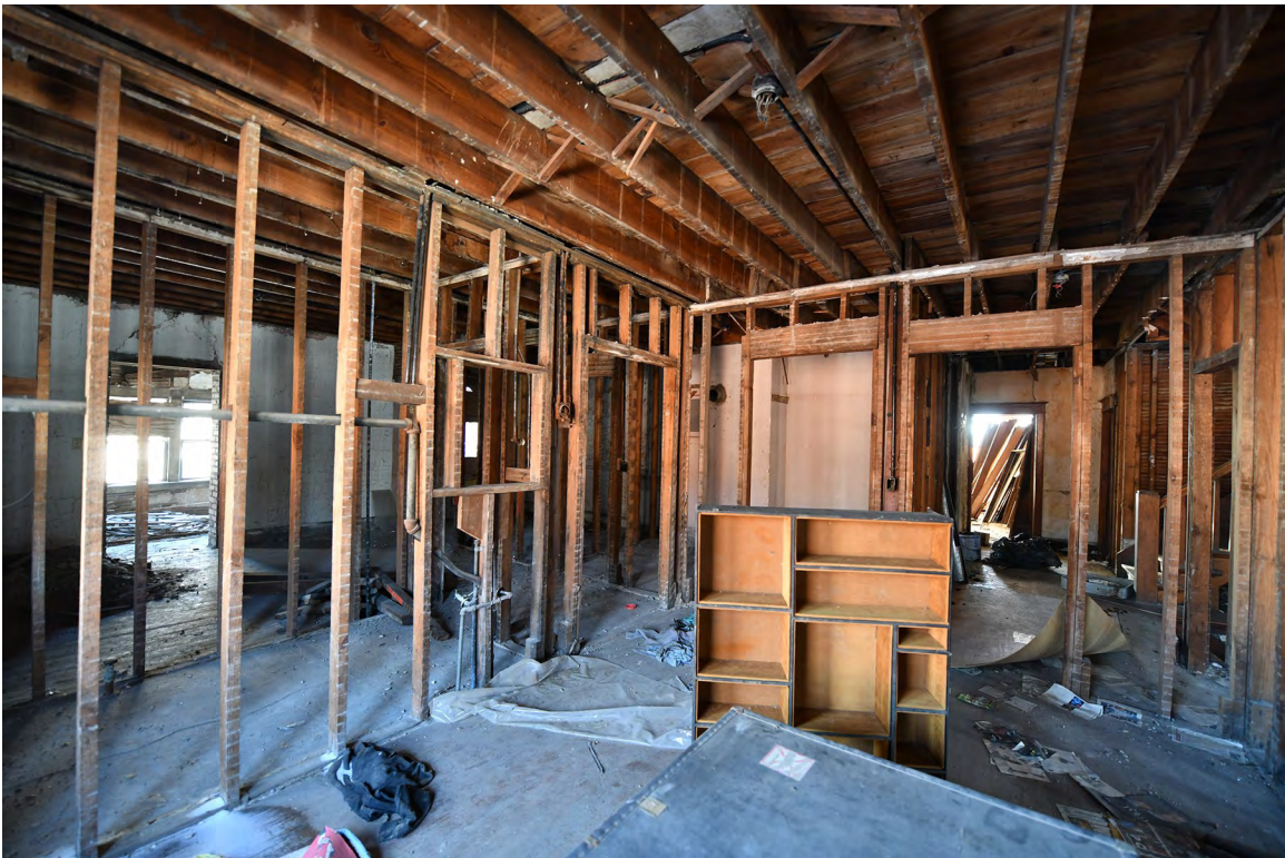
18: Interior, 2nd floor, apartment living room, view SE.
