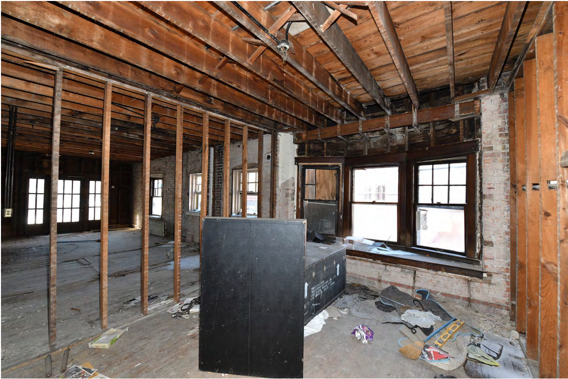
17: Interior, 2nd floor, apartment living room, view NW.
