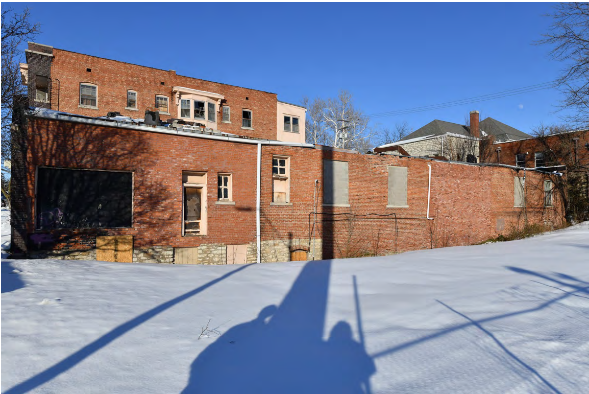
08: Exterior, south elevation (background, partially obstructed), view N.
