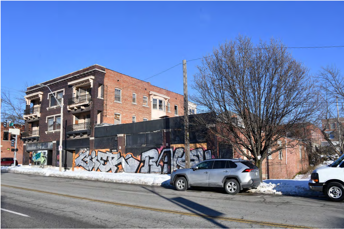
07: Exterior, southwest corner, view NE.
