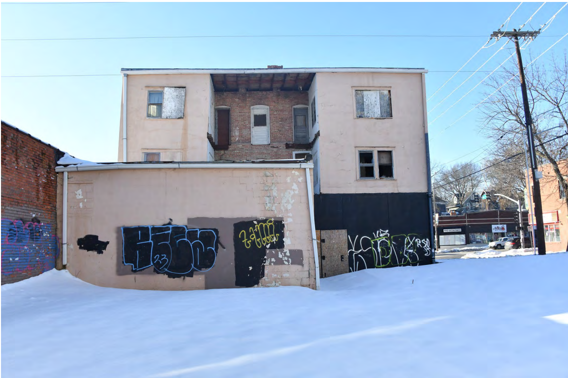
06: Exterior, east elevation, view W.
