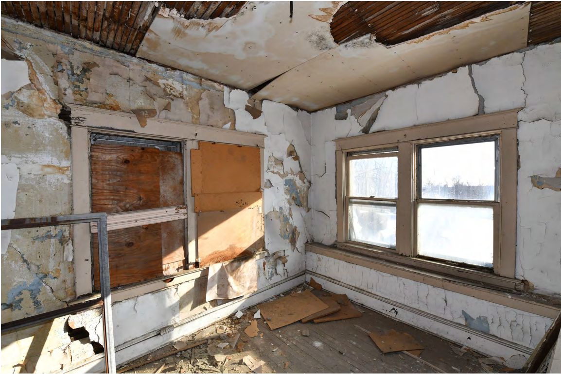
19: Interior, 2nd floor, rear sun room, view SE.
