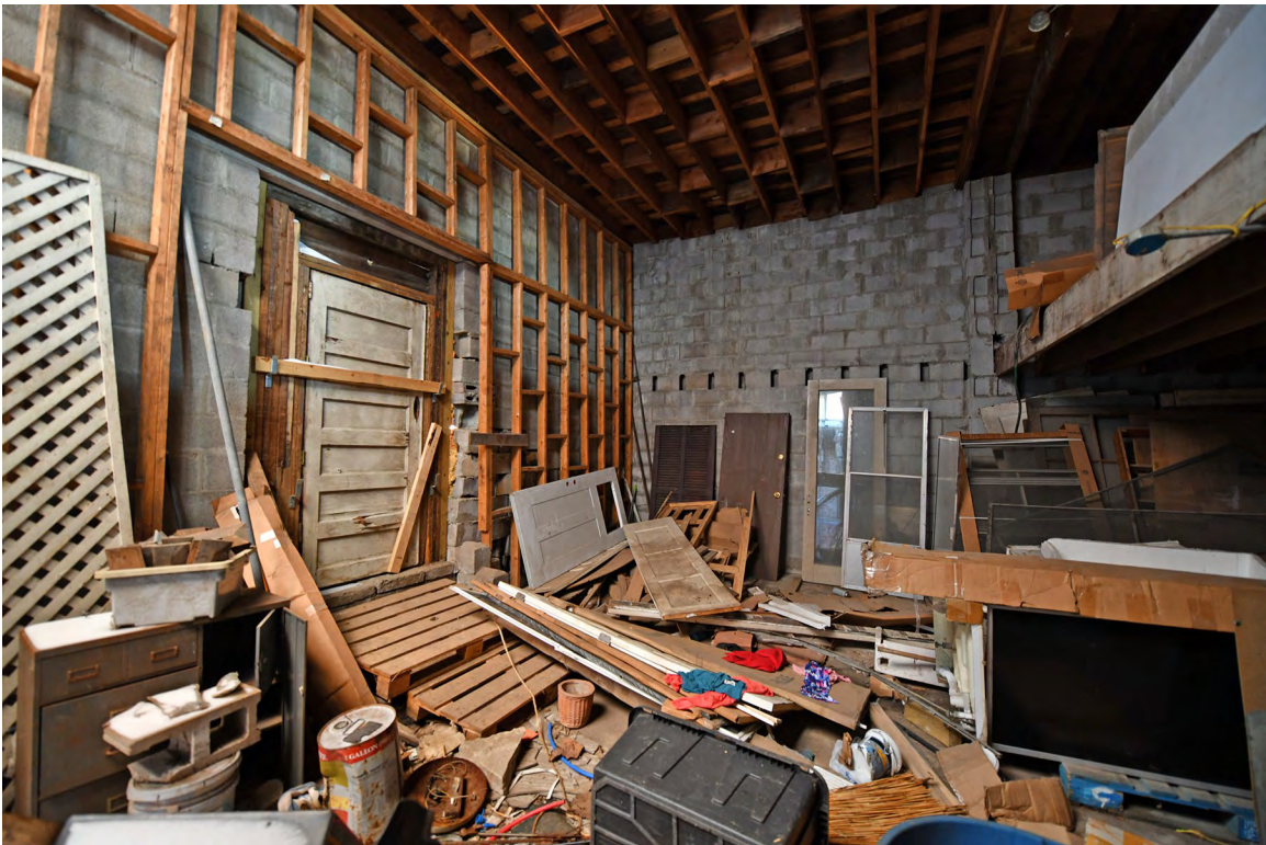
12: Interior, non-historic addition, view NE.
