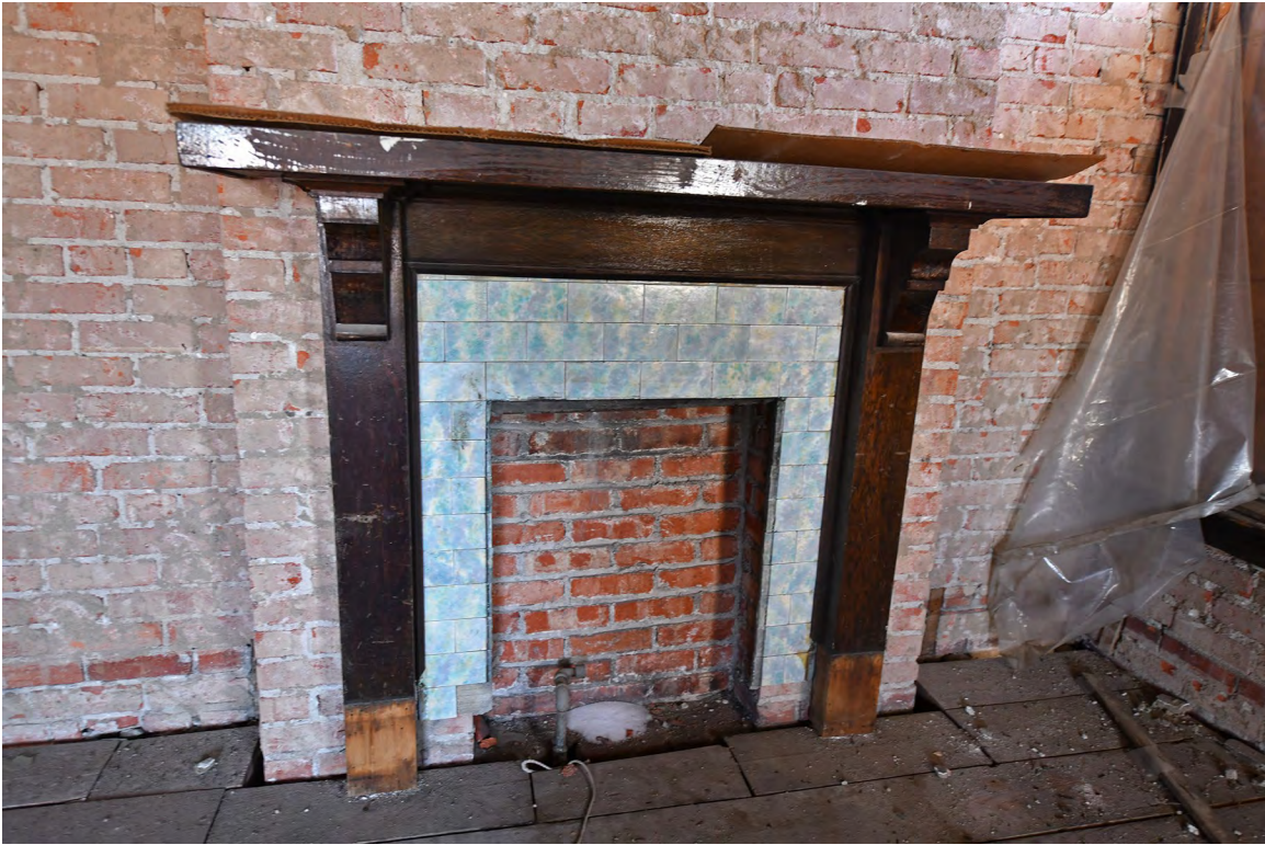
21: Interior, 3rd floor, fireplace detail, view S.
