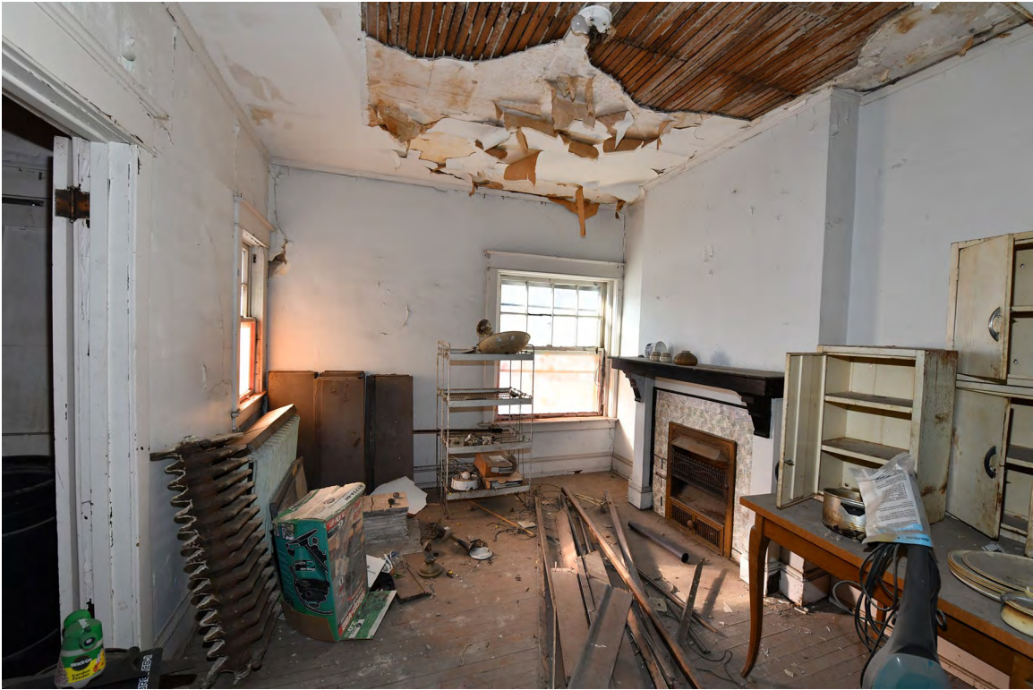
15: Interior, 2nd floor, apartment living room, view NW.
