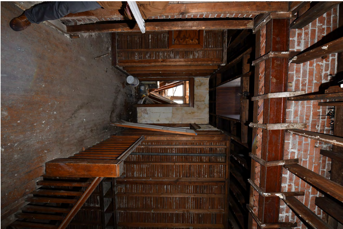
14: Interior, 3rd floor, corridor, view S.
