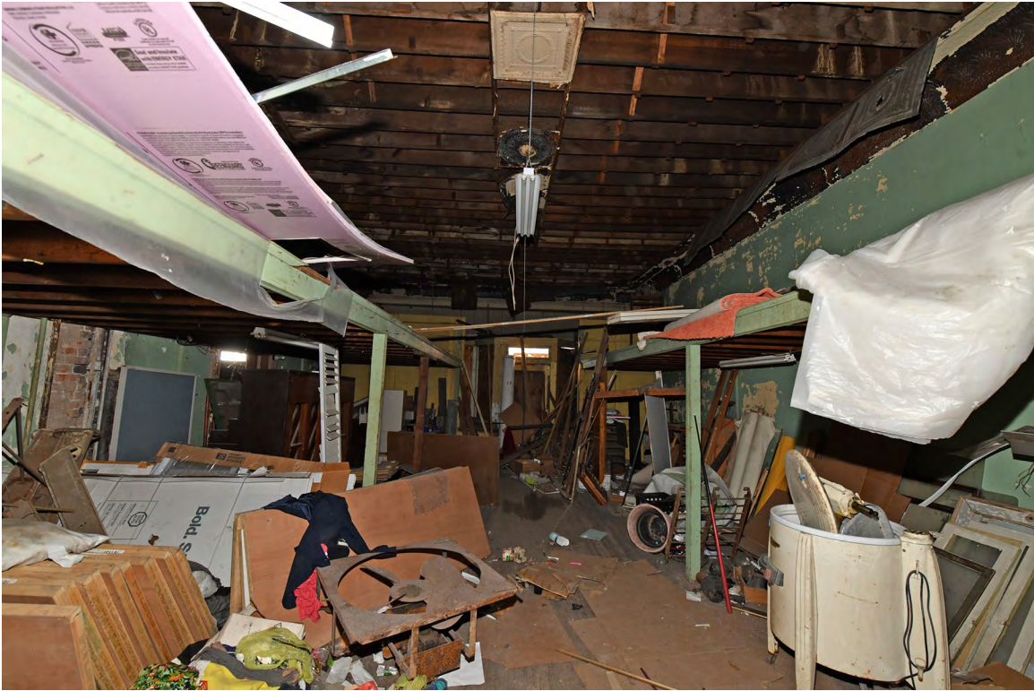
11: Interior, 1st floor, south commercial space, looking from center, view W.
