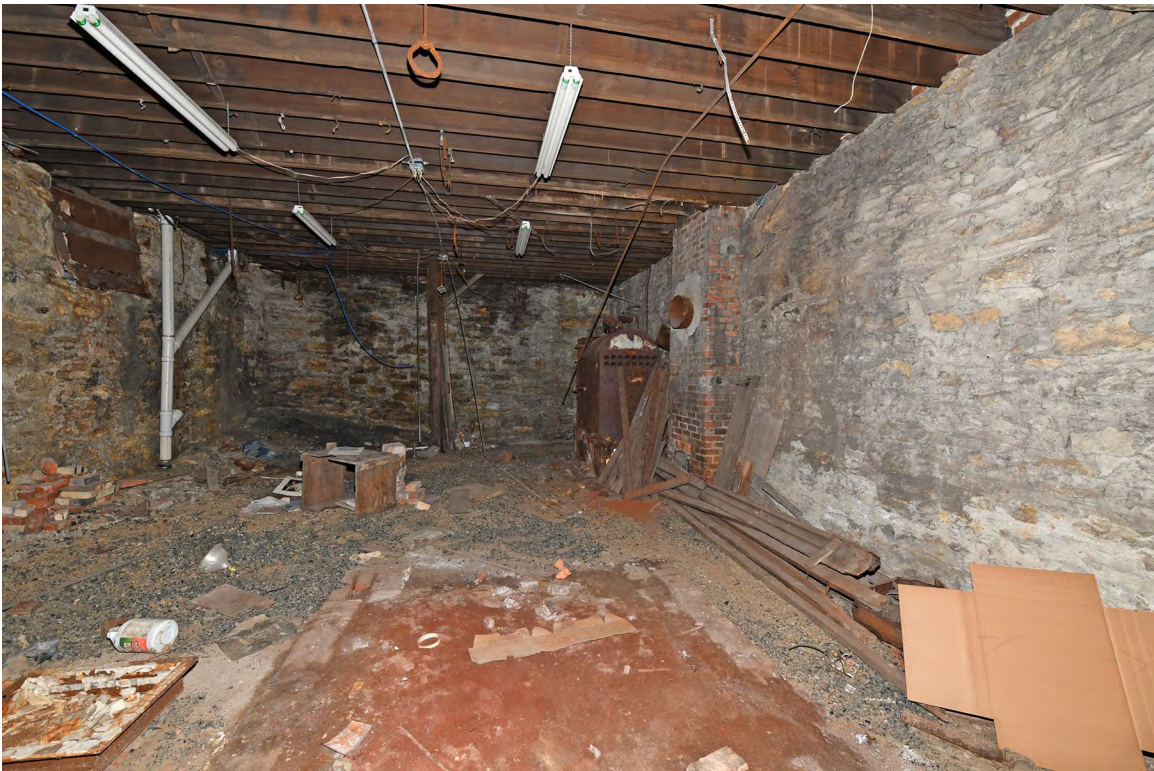
22: Interior, basement, north half, view E.
