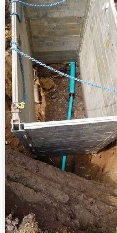
An open cut service lateral repair.
