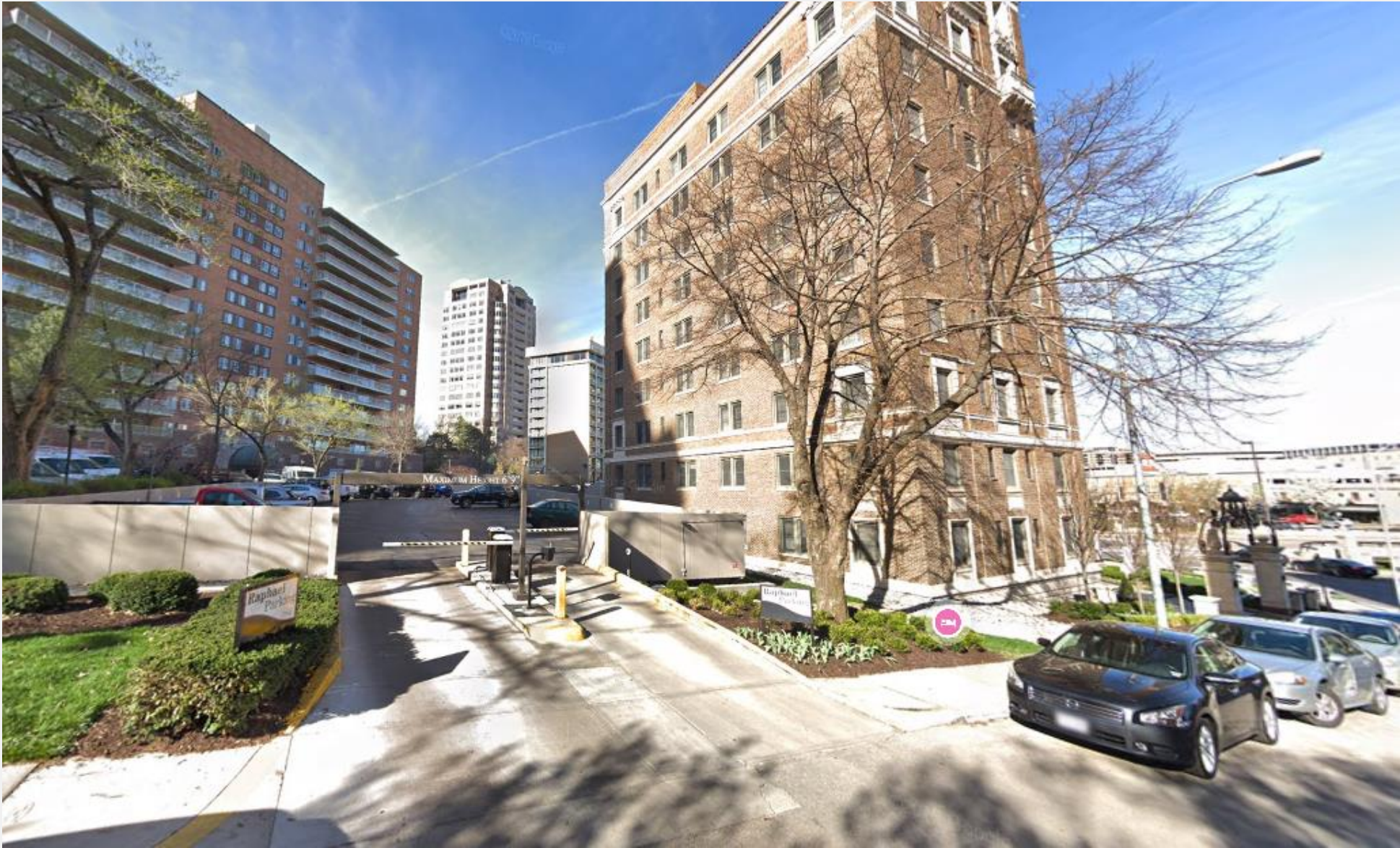
View towards east side of subject site. Entrance to existing parking off W 48 th St.
