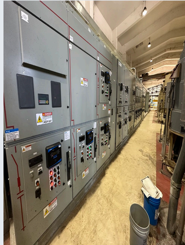
New Electrical Switchgear Equipment
