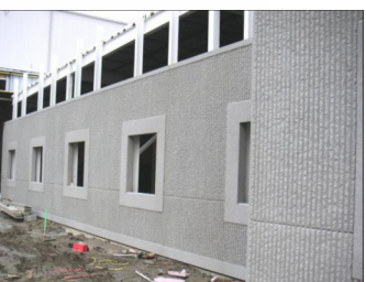
PRECAST FORMLINER PANEL
