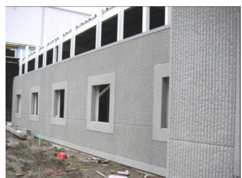
PRECAST FORMLINER PANEL
