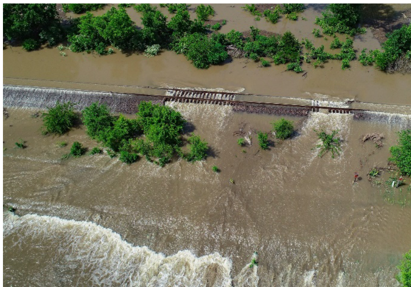
Figure 4.10.1: Breached Levee in Levasy, Missouri
