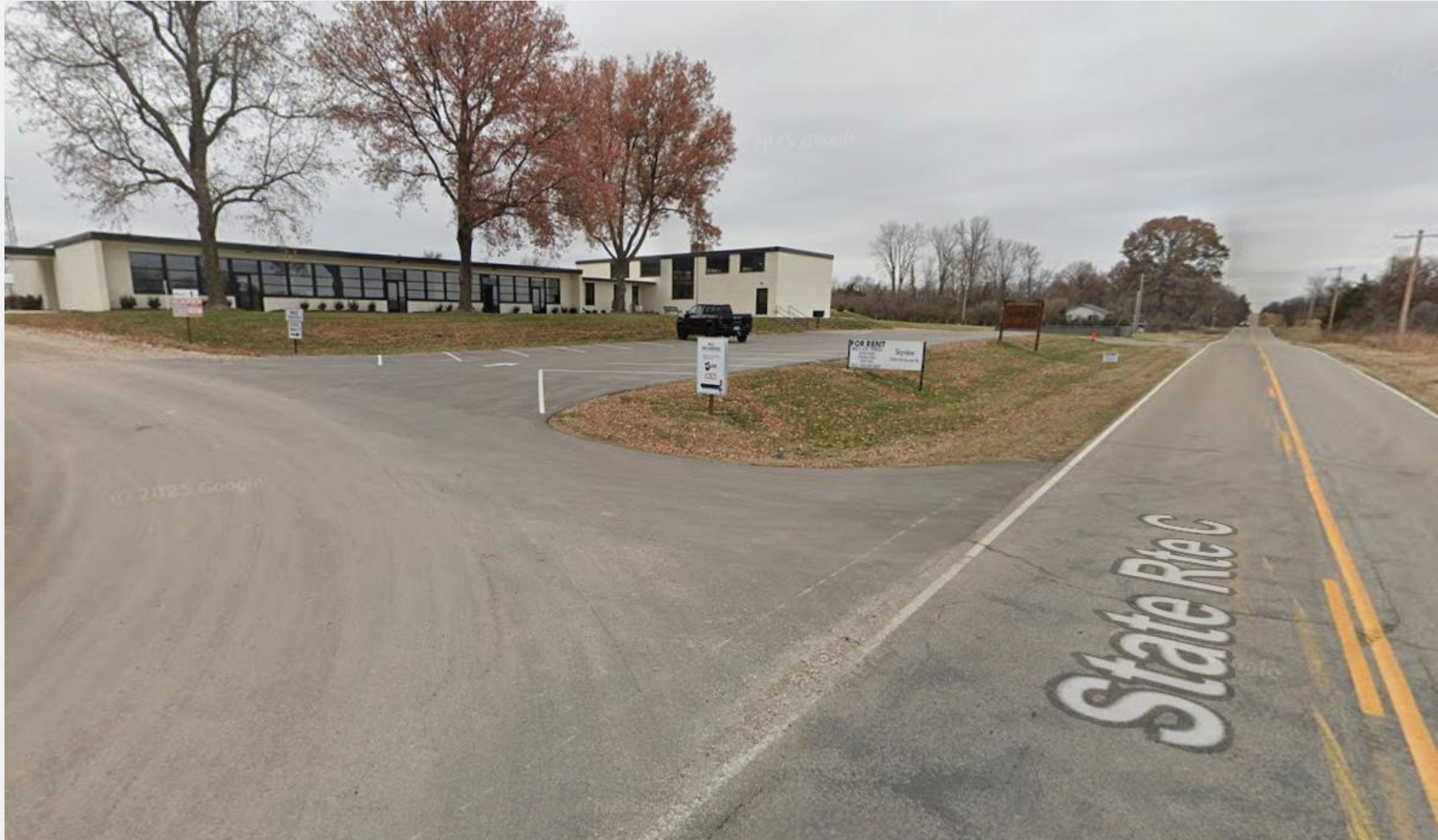
View of site from NW Skyview Ave
