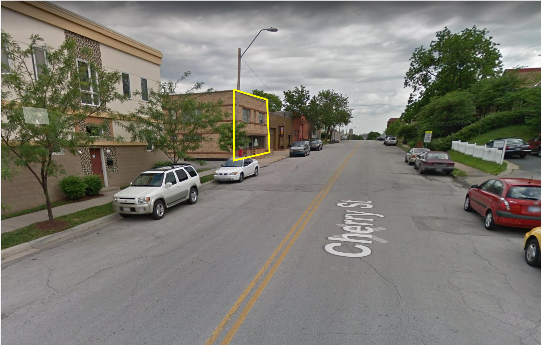
View looking north on Cherry St. Subject site on left
