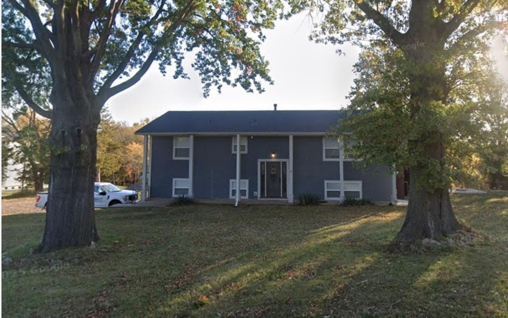
Existing Single-Family House
