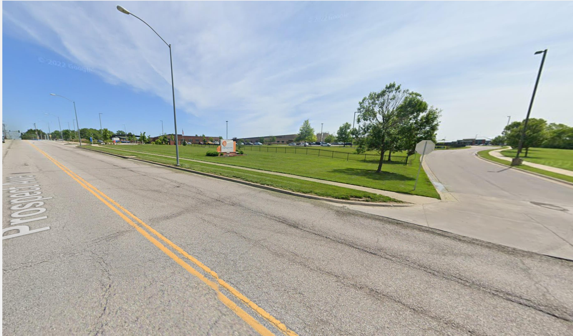
View northeast towards site from Prospect Ave
