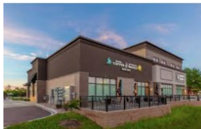
Canopy Canopy is 8'-0" or higher Above walkway Windows Street facing façade windows are encouraged
