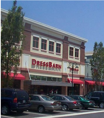
Buildings should integrate elements such as awnings to enhance the street edge.
