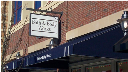
Low-scale signs, such as the wall sign shown above, are preferred within new retail areas.
