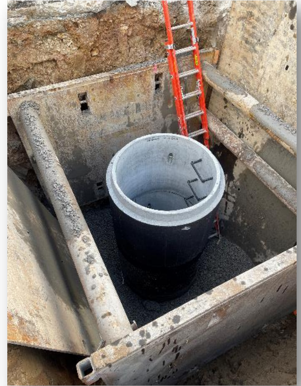
Sewer Manhole Replacement
