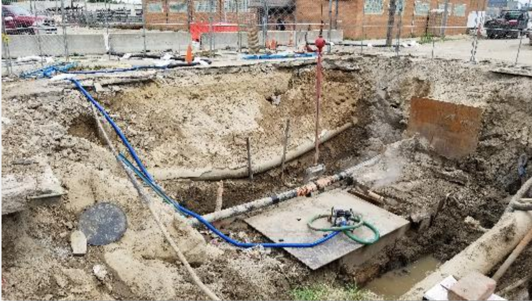
Emergency 18-inch Sewer Repair at 1700 Guinotte Avenue
