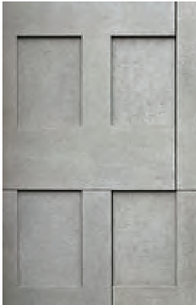
ARCHITECTURAL C.I.P CONCRETE WARM GREY
