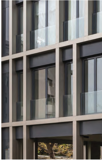
EXPRESSED GRID - METAL PANEL WARM GREY - (TUBELITE OR SIMILAR)
