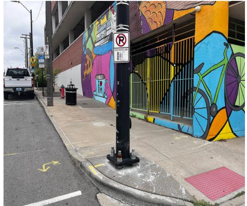
Third & Walnut Streets – Sidewalk Replacement w/ADA
