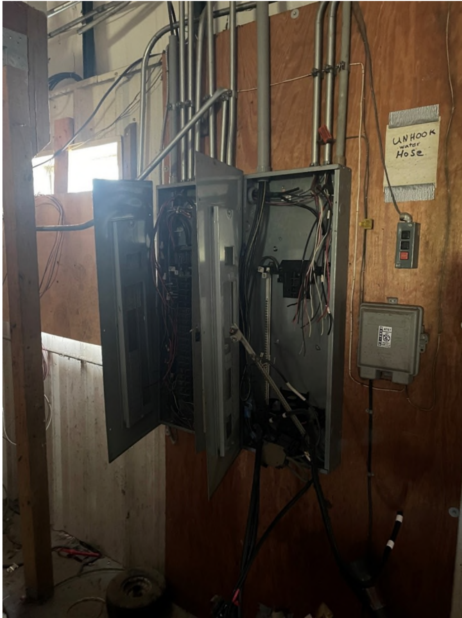
Destroyed electrical box from trespassers.
