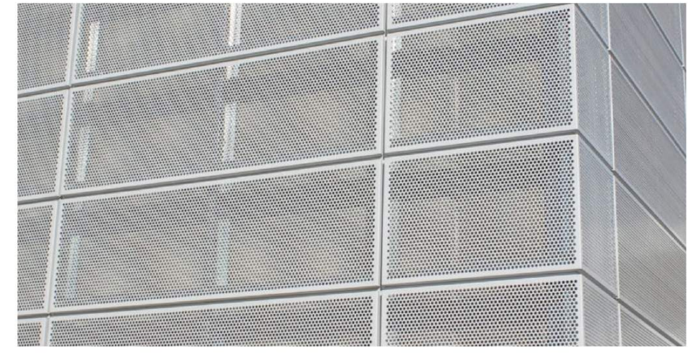
PERFORATED METAL SCREEN WALL / SUN SCREEN
