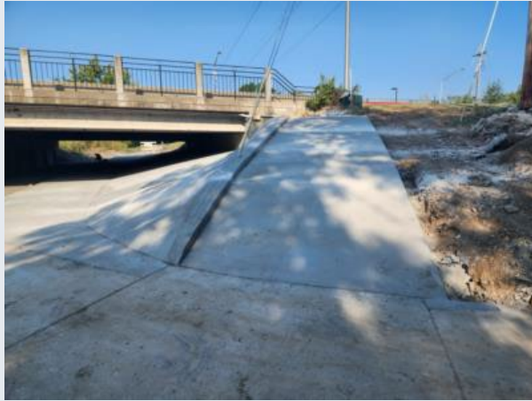
Concrete slope protection and trail replacement on the north end of the Wornall Bridge
