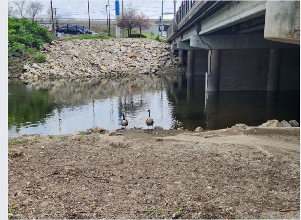
East side of Wornall Road Bridge
