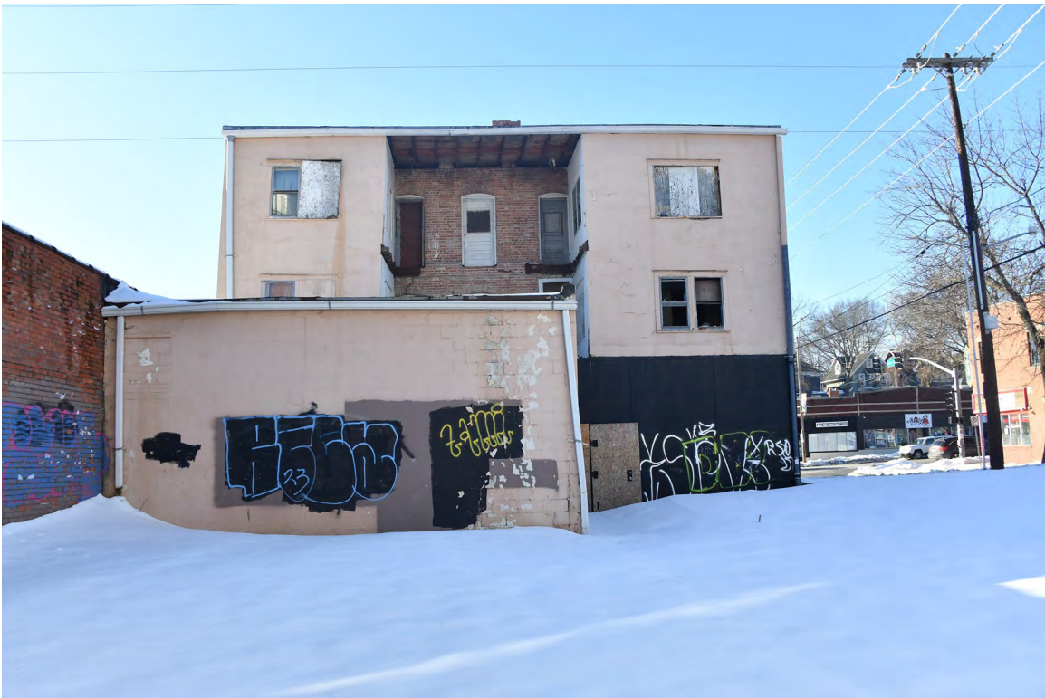
06: Exterior, east elevation, view W.
