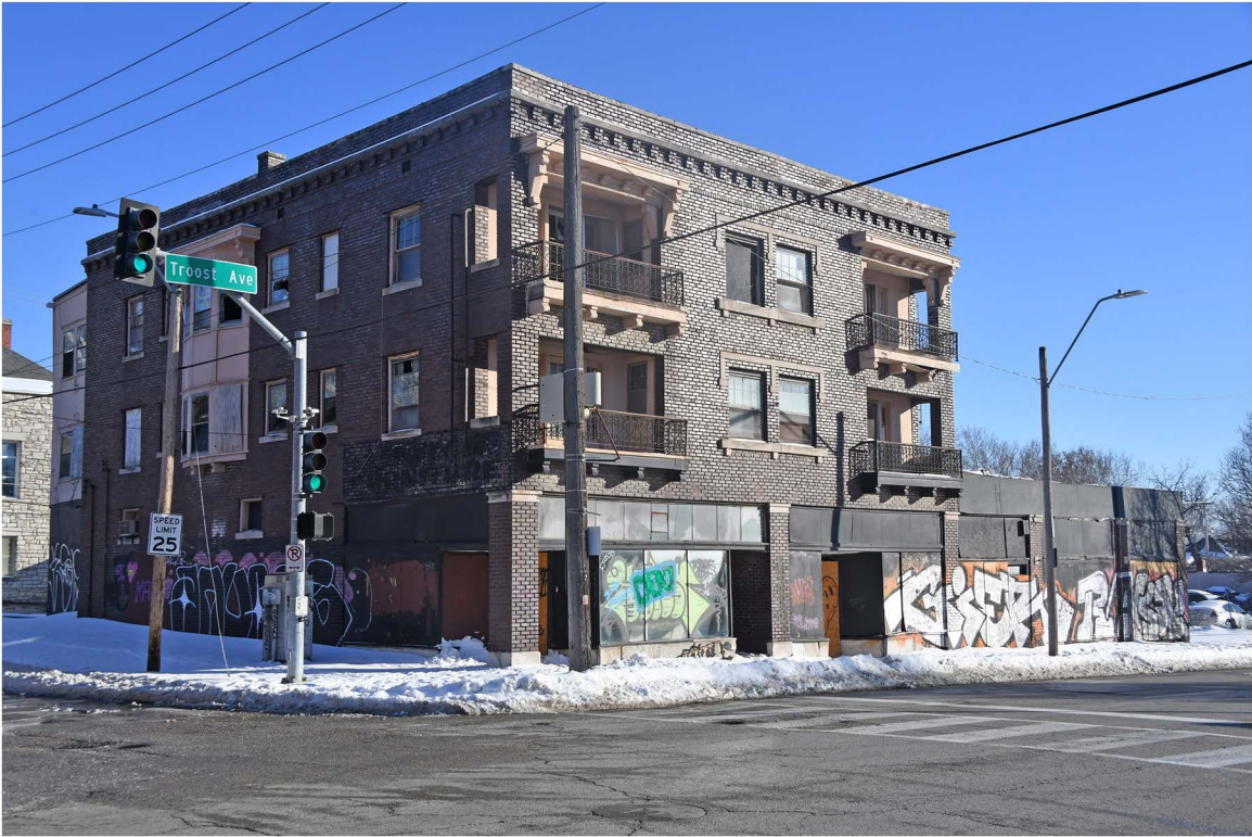
01: Exterior, northwest corner, view SE.
