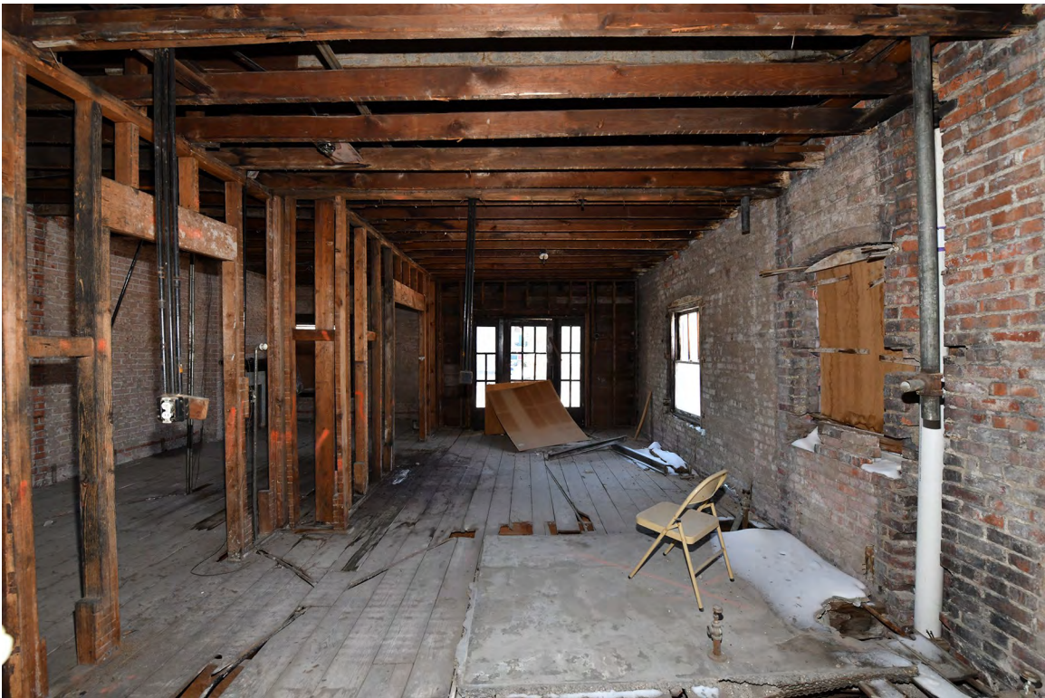
20: Interior, 3rd floor, apartment, view W.
