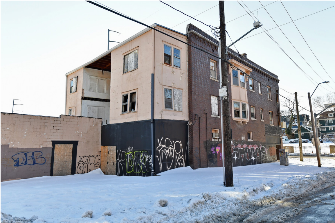
05: Exterior, northeast corner, view SW.
