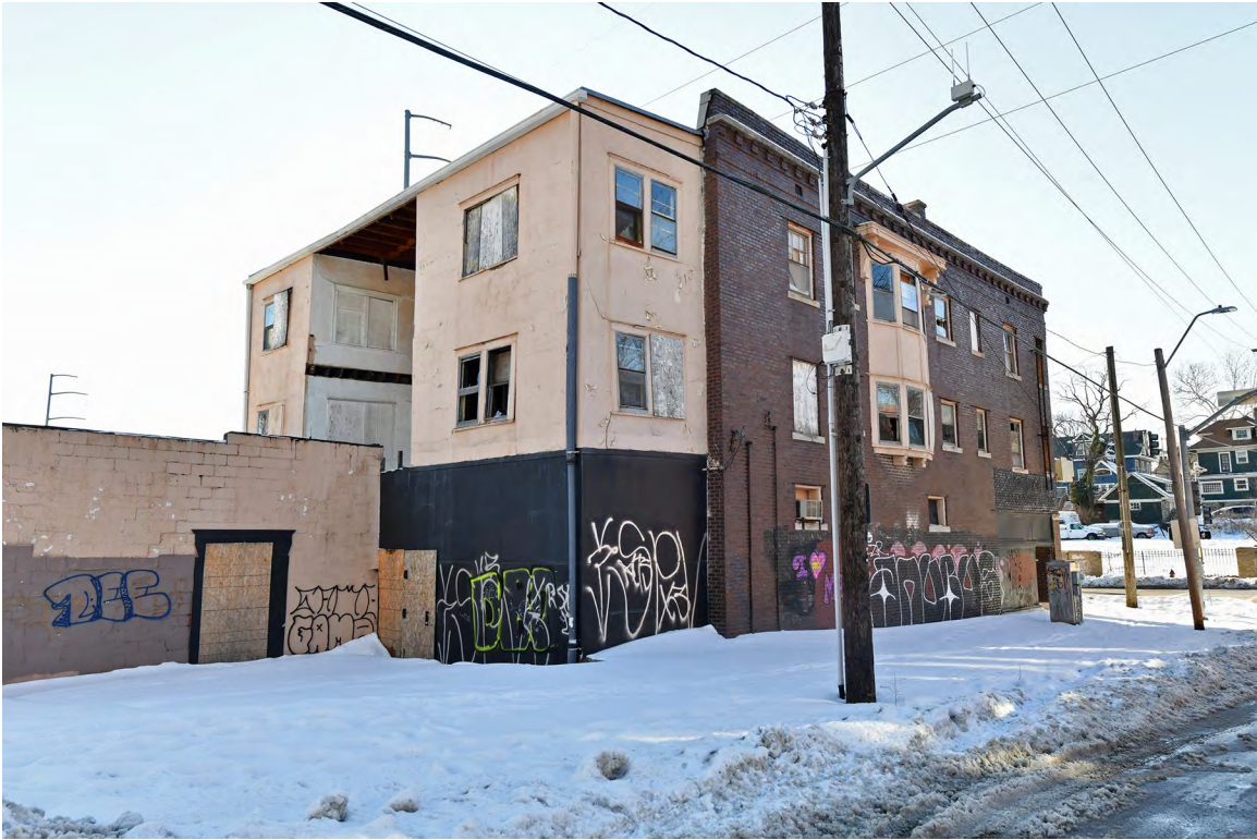
05: Exterior, northeast corner, view SW.
