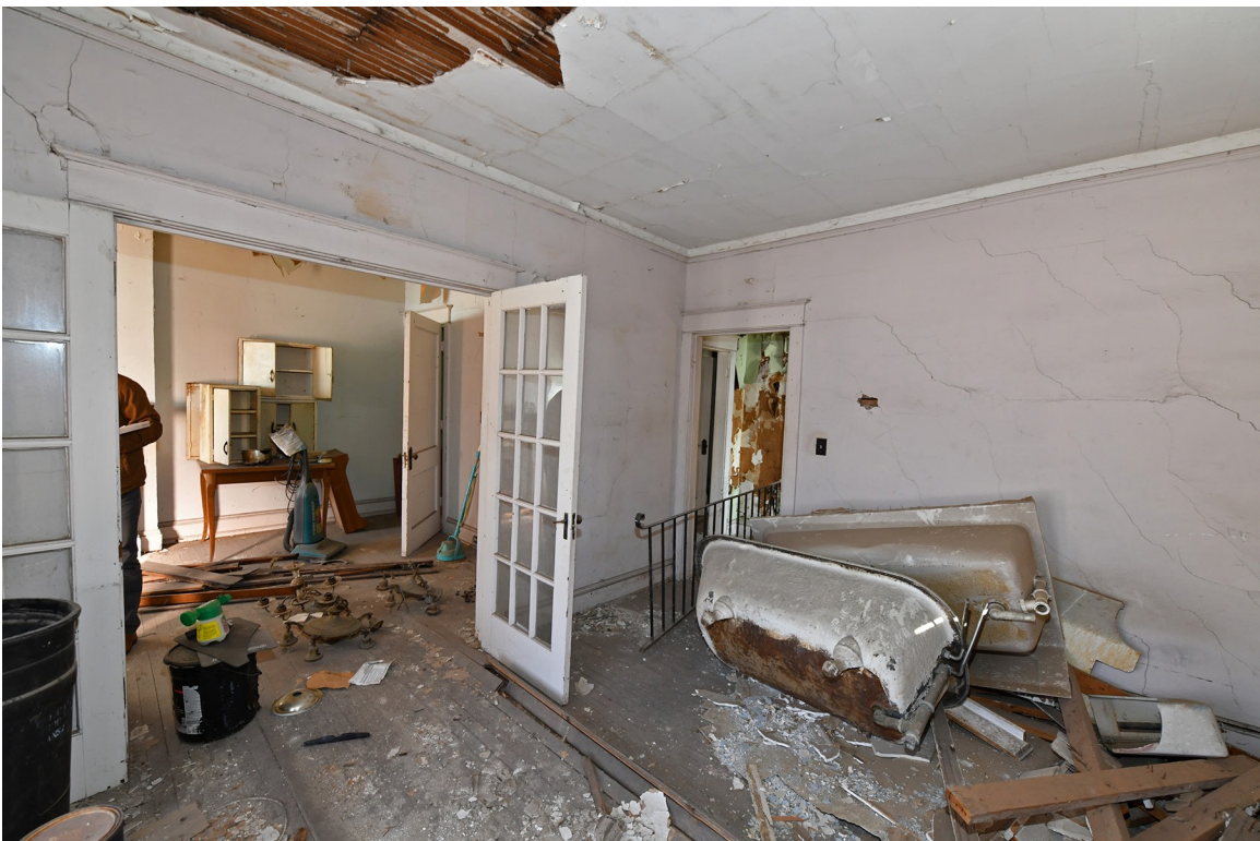
16: Interior, 2nd floor, apartment bedroom, view NE.
