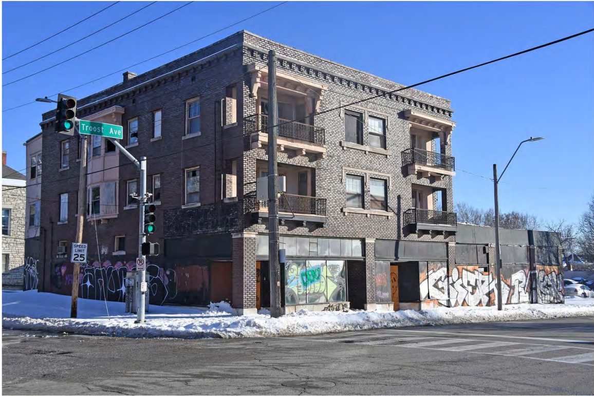
01: Exterior, northwest corner, view SE.
