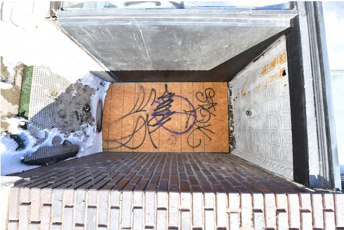
04: Exterior, west elevation, apartment entrance, view E.
