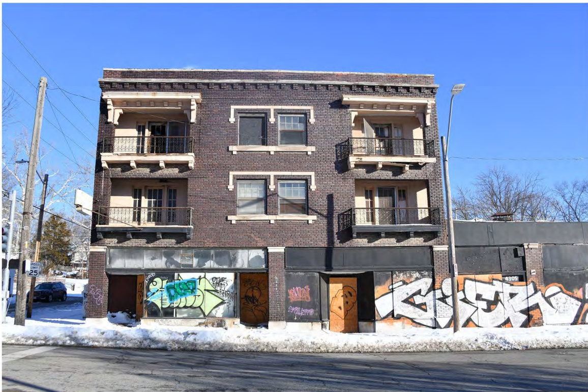
02: Exterior, west (primary) elevation, view E.
