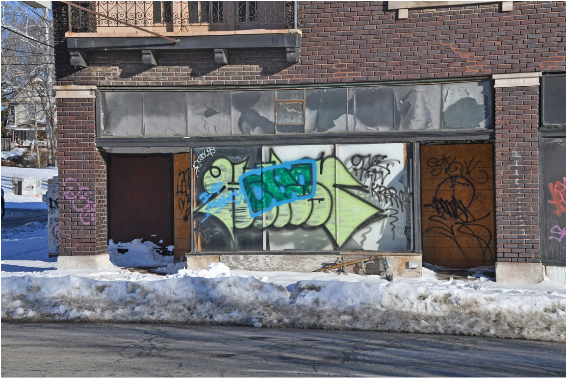
03: Exterior, west elevation, north storefront, view E.
