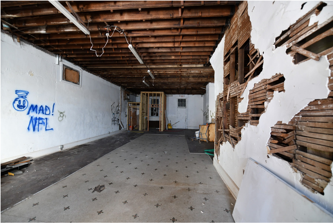
09: Interior, 1st floor, north commercial space, looking from entrance, view E.
