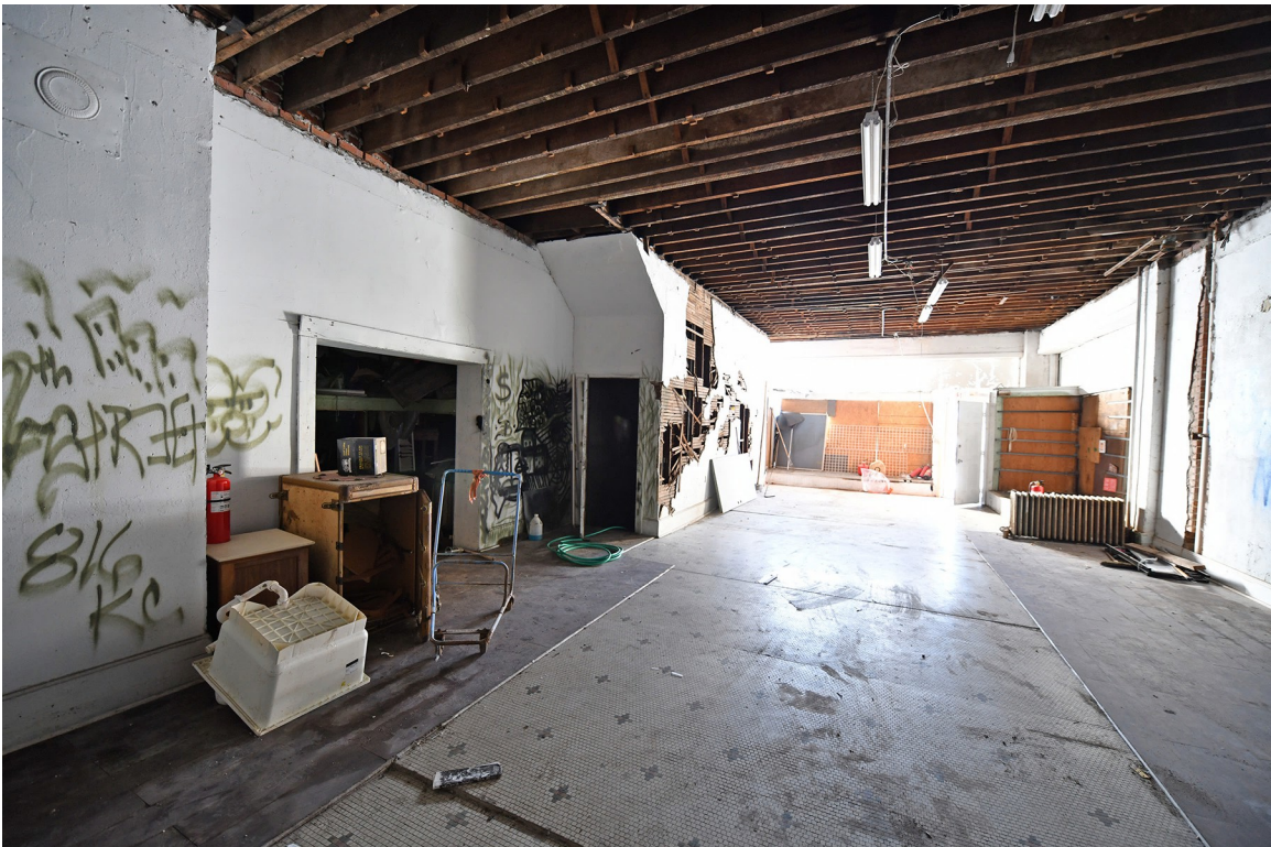
10: Interior, 1st floor, north commercial space, looking from back, view W.
