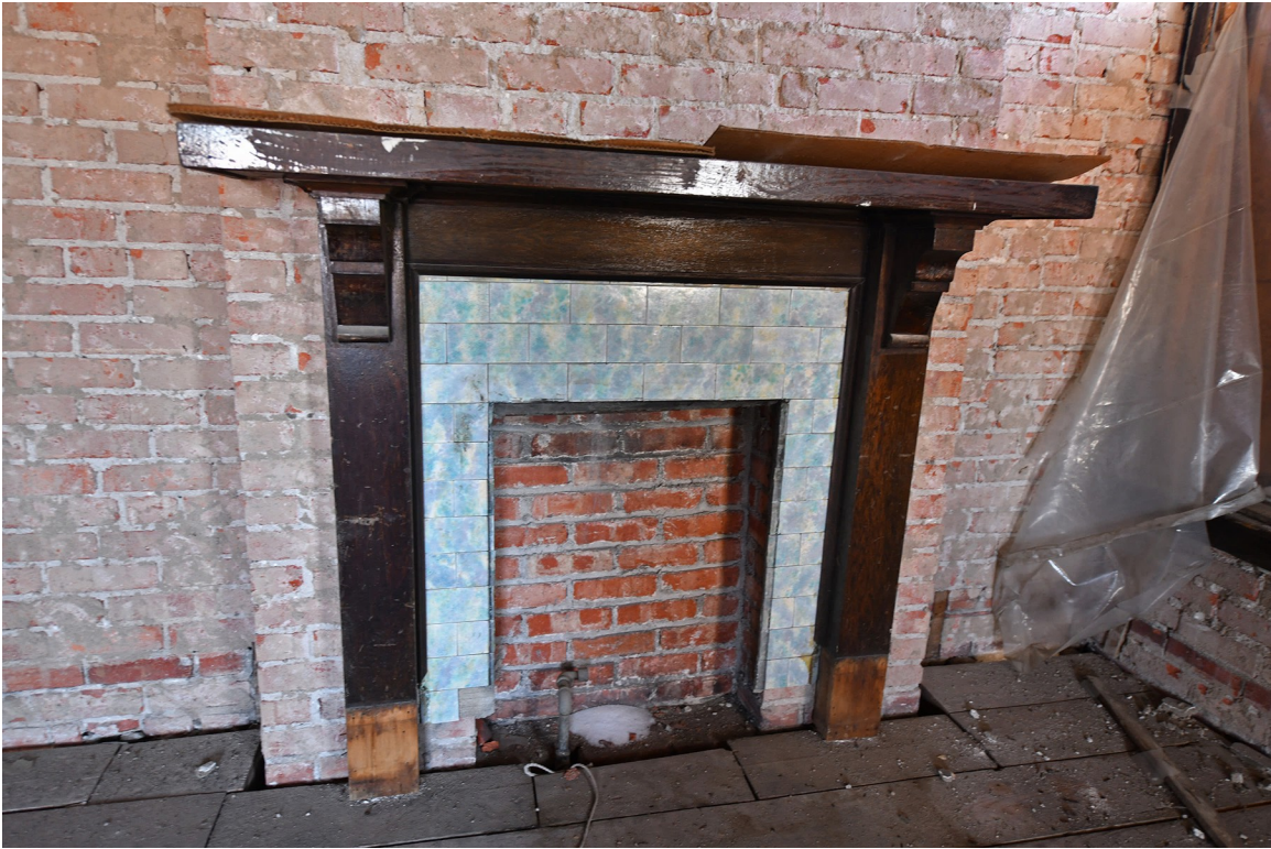
21: Interior, 3rd floor, fireplace detail, view S.
