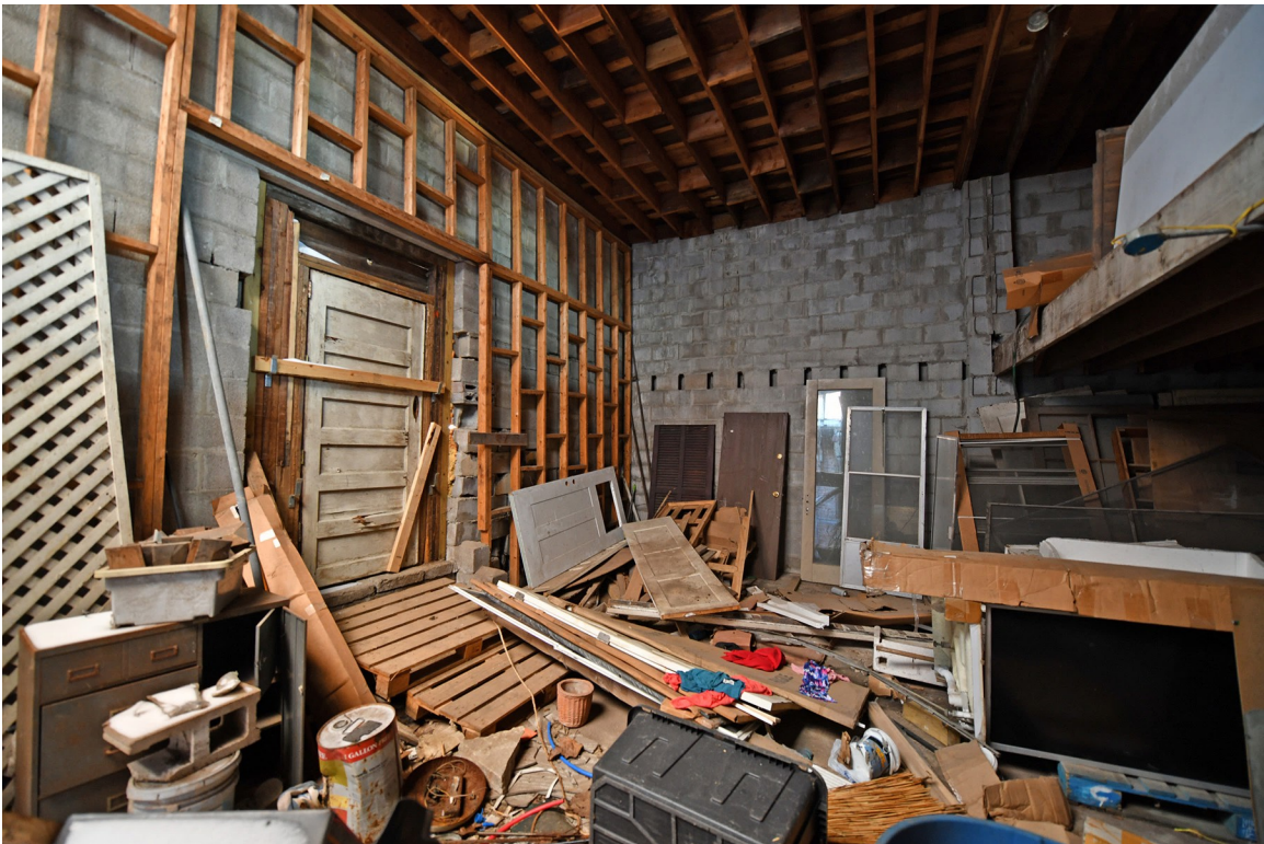
12: Interior, non-historic addition, view NE.
