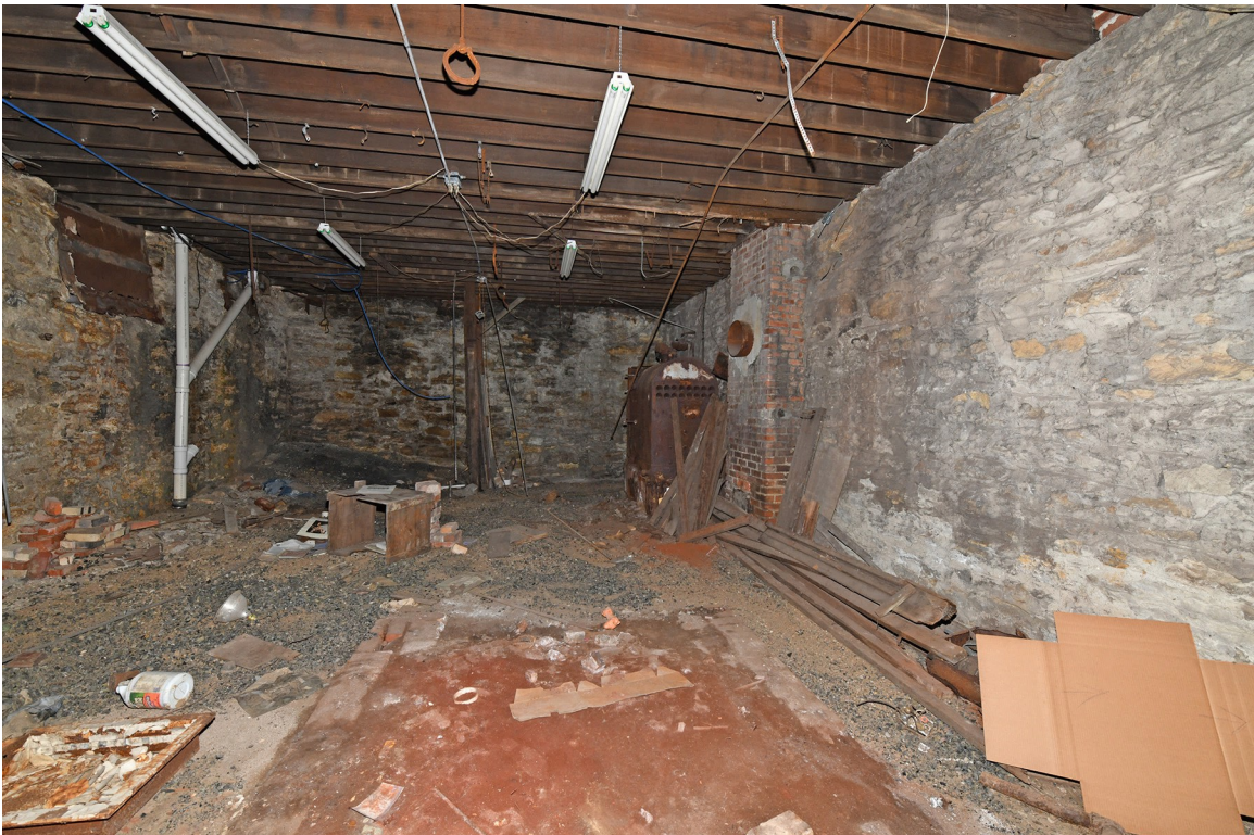
22: Interior, basement, north half, view E.
