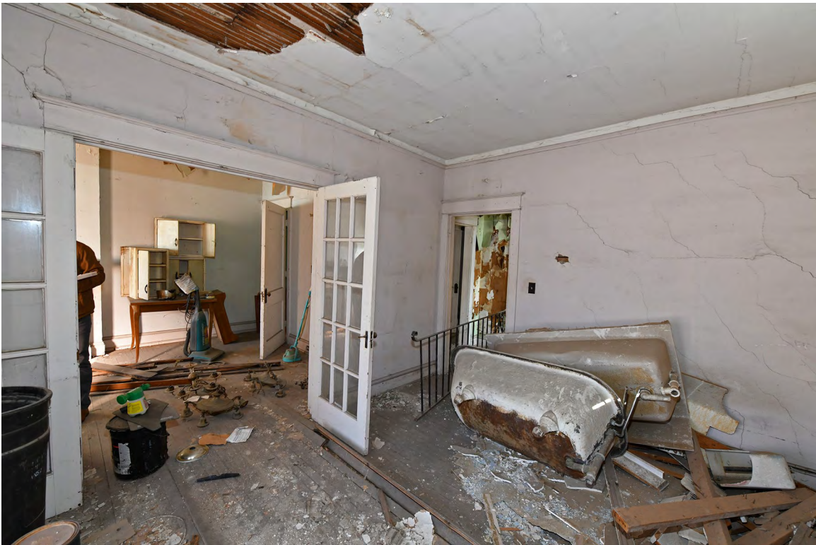
16: Interior, 2nd floor, apartment bedroom, view NE.
