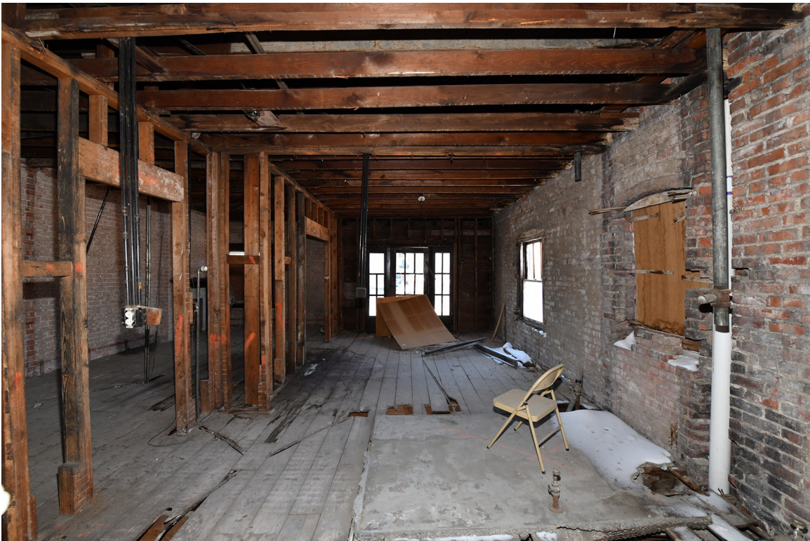
20: Interior, 3rd floor, apartment, view W.
