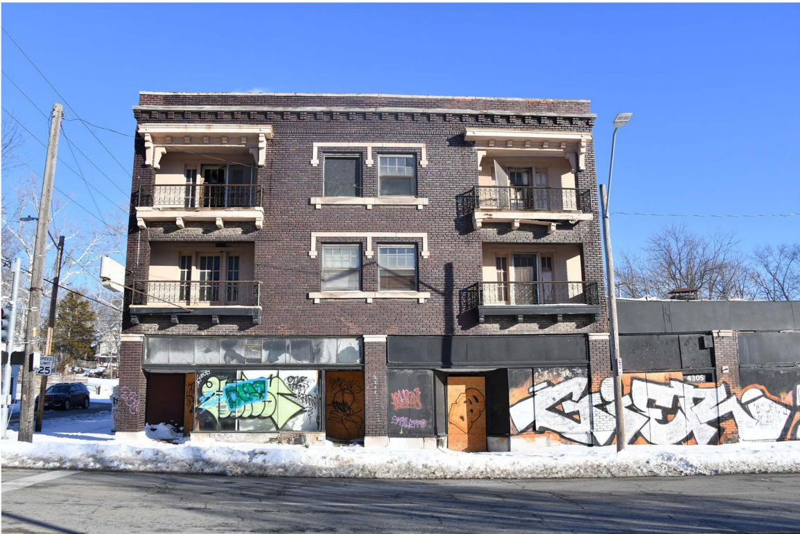
02: Exterior, west (primary) elevation, view E.
