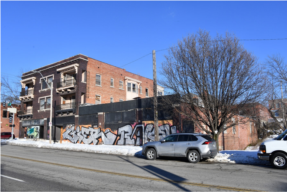
07: Exterior, southwest corner, view NE.
