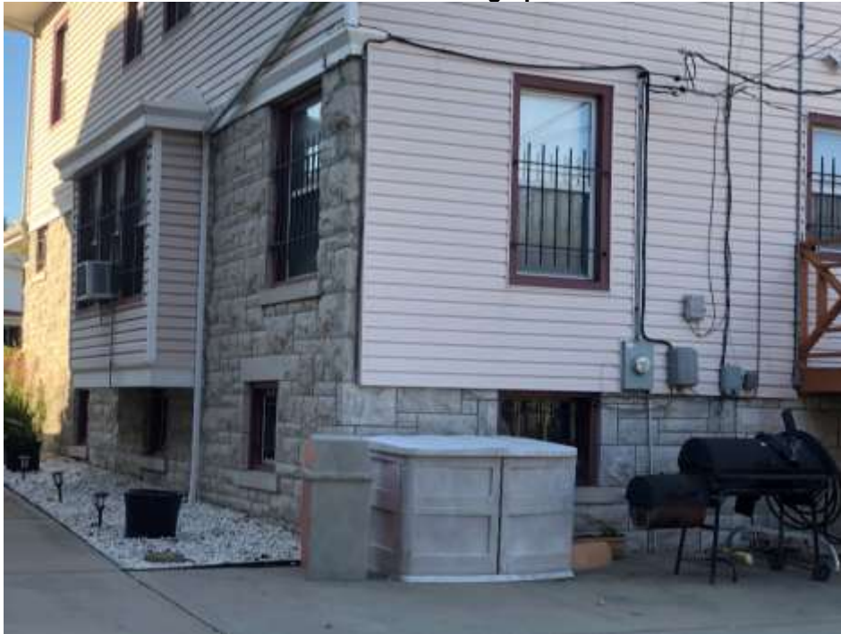
Rear and East Facades
