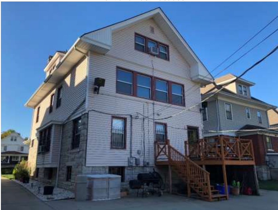
Rear (North) and East Façade
