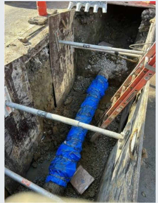
Replacement of a Cast Iron with Ductile Iron Pipe
