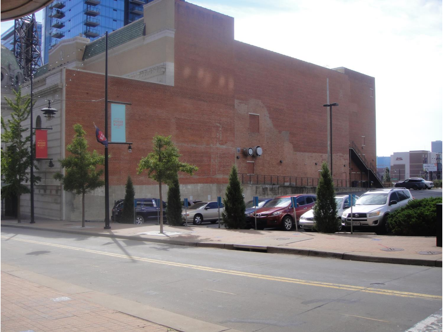
Photo 2 – Block 138. View of southwest corner of Baltimore Avenue and 14 th Street. Note B & B Mainstreet Theater to the left (not located within the Redevelopment Area).
