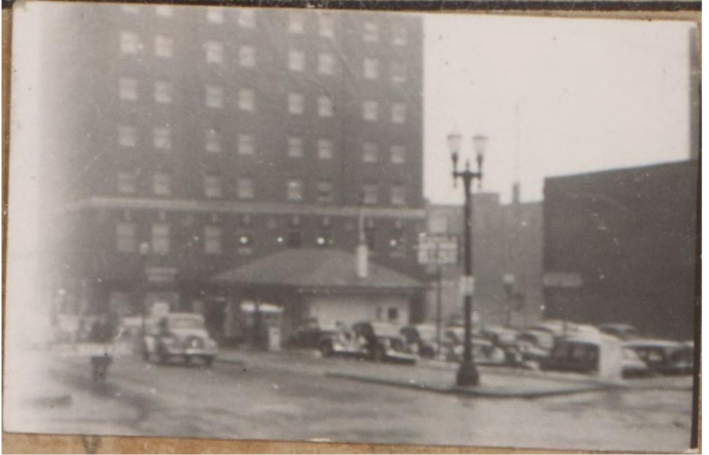
Figure 12 - 1940 Photograph of the former gas station located on Block 138. Impacts of this facility to the block are unknown. Image courtesy KC Public Library.
