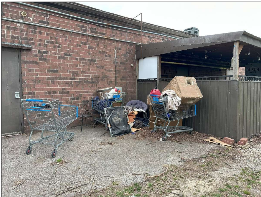
Tiffany Plaza – looking southeast – trash/debris; uneven pavement
