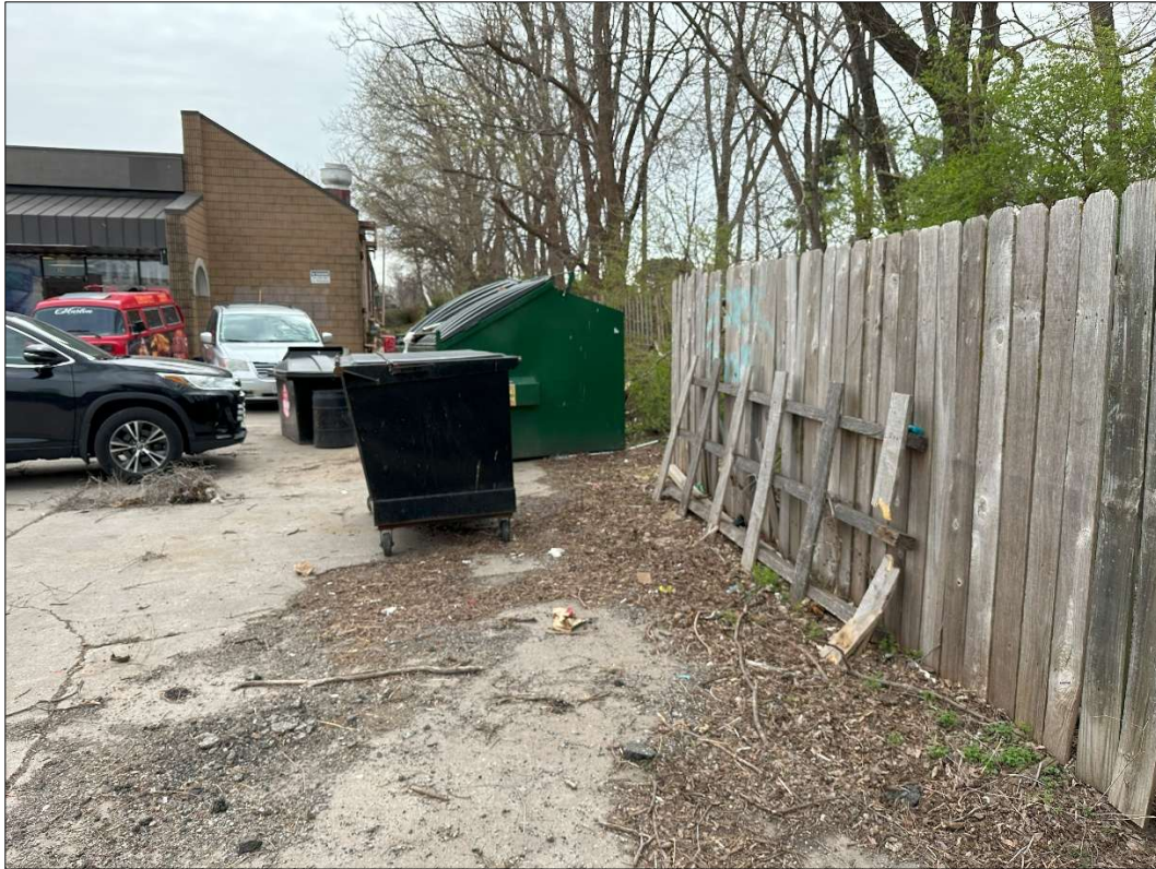
Tiffany Plaza – looking south – deterioration of pavement, fence; unenclosed dumpsters
