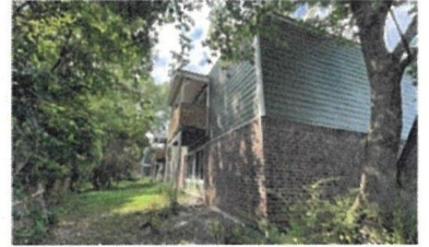
BUILDING 500 SOUTHWEST ELEVATION
