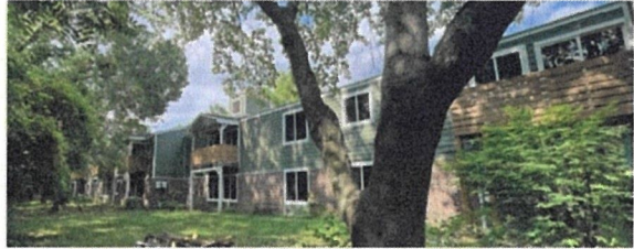
BUILDING 500 SOUTHWEST ELEVATION CONTINUED
