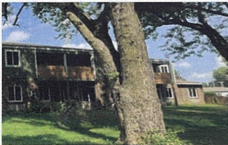
BUILDING 400 SOUTHWEST ELEVATION
