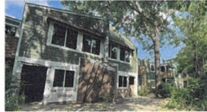
BUILDING 500 SOUTHWEST ELEVATION CONTINUED
