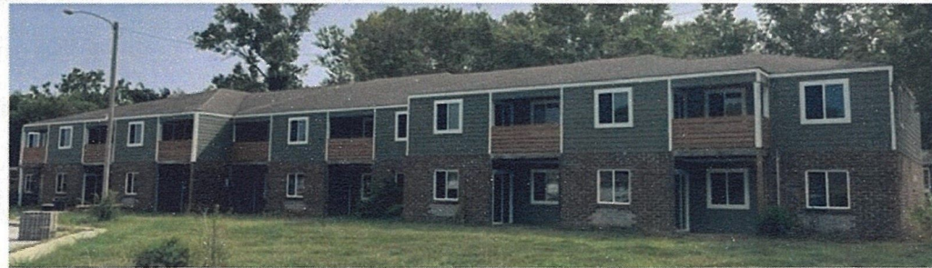
BUILDING 400 NORTHEAST ELEVATION
