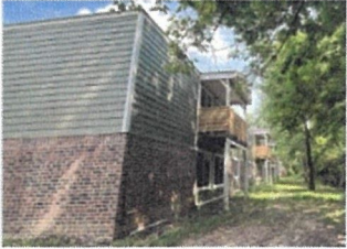
BUILDING 500 SOUTHWEST ELEVATION CONTINUED
