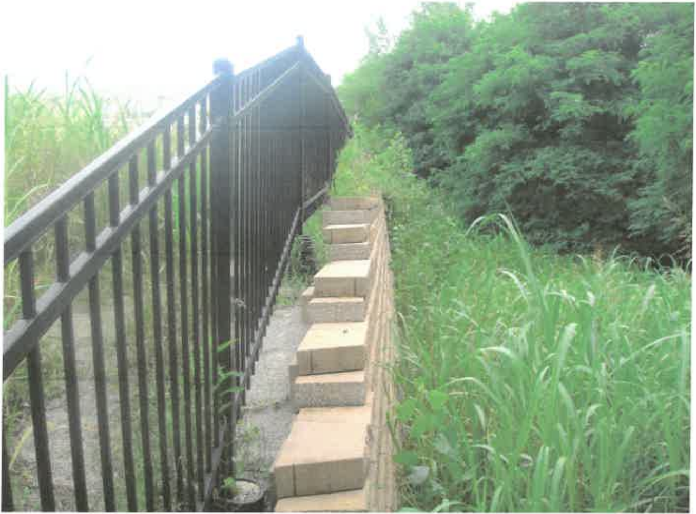
Photo 7 - Retaining wall along eastern property boundary. Wall is approximately 20' in height at this location.
