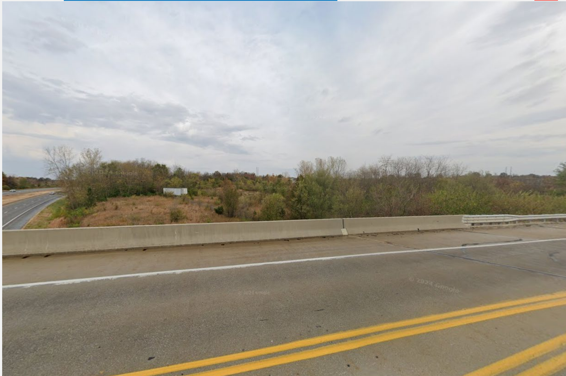
Looking north on NE Barry Rd. (Oct 2024)
