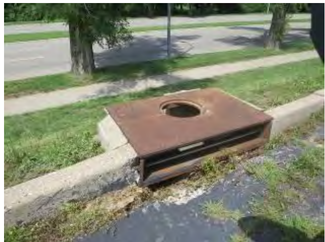
Deteriorating Sewer Inlet At 3011 Swope Parkway
