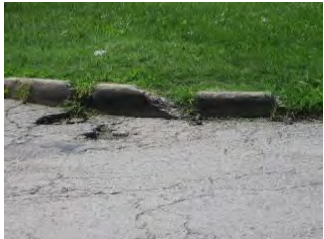
Deteriorated Curbs Along Agnes Avenue
