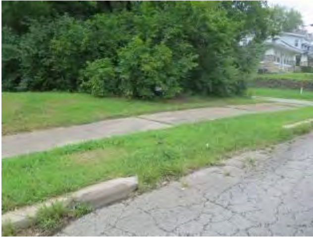
Deteriorating Curbs & Lack Of Gutters – College Ave.
