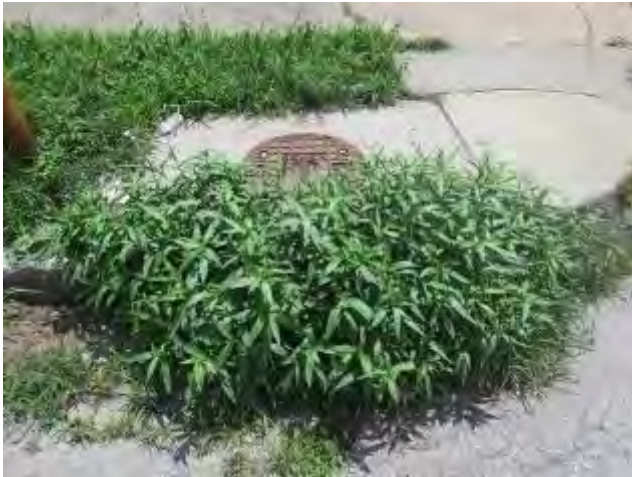
Clogged Sewer Inlet Along E 49 th Street
