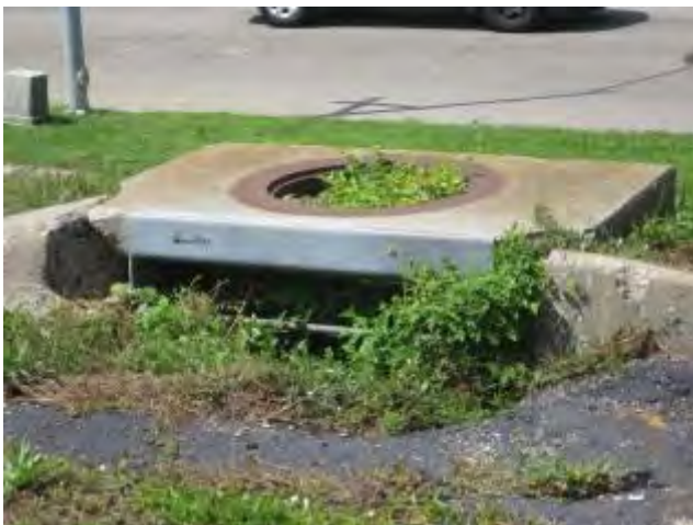
Clogged Sewer Inlet At 3011 Swope Parkway
