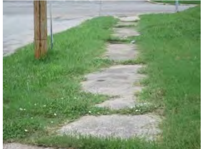
Deteriorating/Unsafe Sidewalk Along Agnes Avenue
