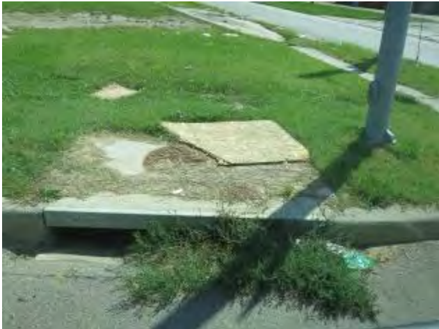
Clogged Sewer Inlet Along Swope Parkway
