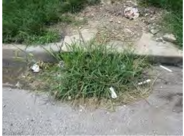
Clogged Sewer Inlet Along Chestnut Avenue
