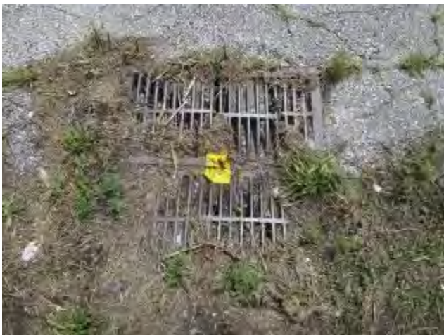
Clogged Sewer Inlet At 2801 Swope Parkway
