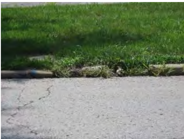
Deteriorated Curbs Along Agnes Avenue
