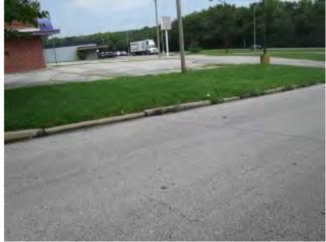
Deteriorating Curbs Along College Avenue
