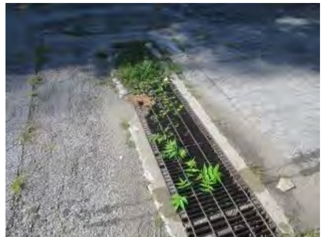
Clogged Drainage Grate At 2915 Swope Parkway
