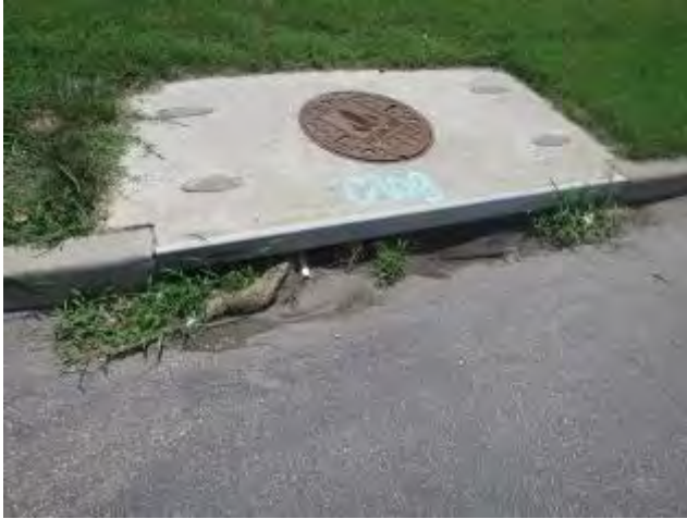
Clogged Sewer Inlet Along Swope Parkway
