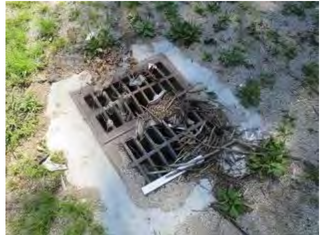
Clogged Sewer Inlet At 3011 Swope Parkway
