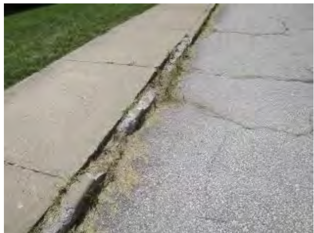
Deteriorated Curbs At 2801 Swope Parkway
