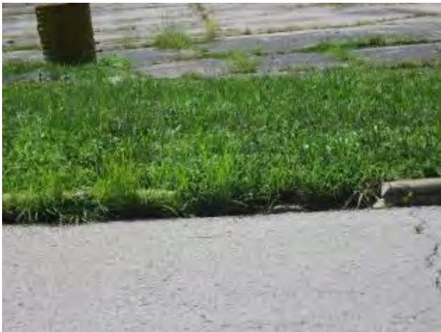
Deteriorated Curbs Along Agnes Avenue
