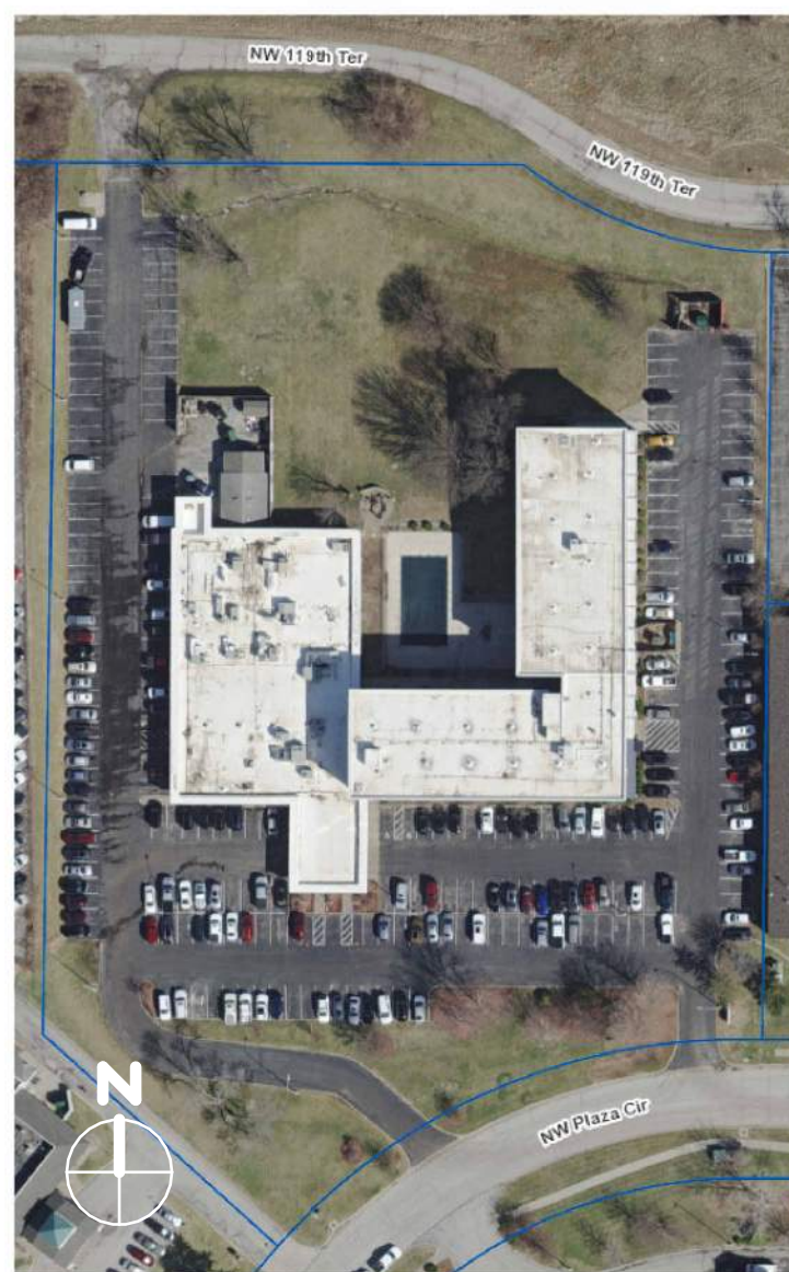
Existing Site View
