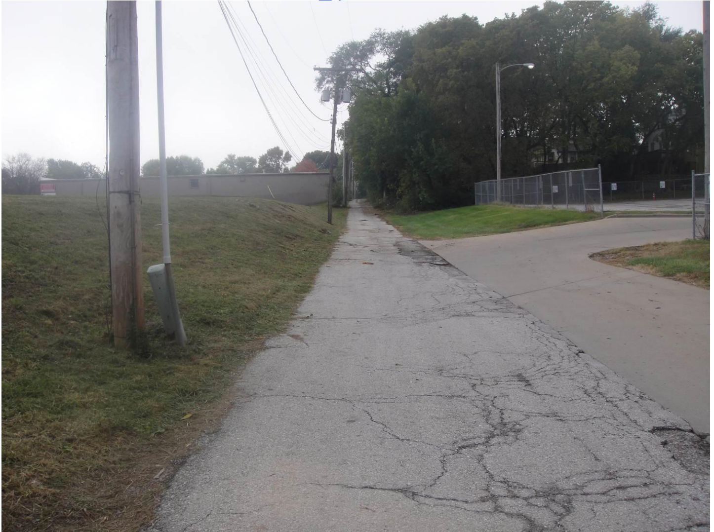
Photo 17 – View south along alleyway. Subject area to left. Note topographic rise of the subject area.
