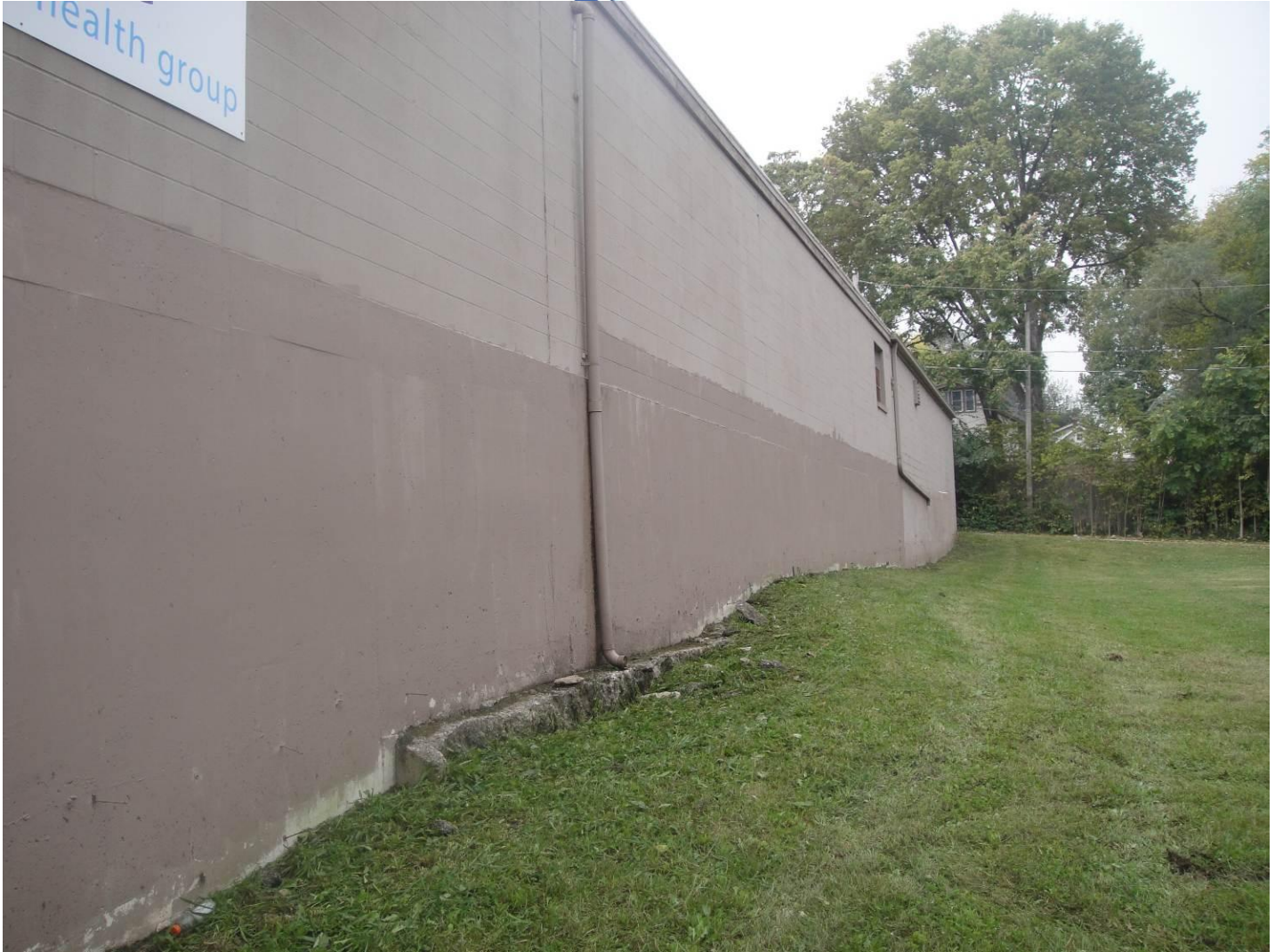
Photo 12 – Exterior wall, north side of 2534 Campbell Street.
