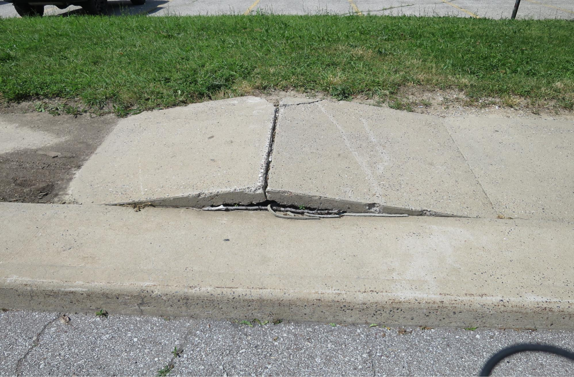
Heaving Concrete Sidewalk North Side Of E 9 th St. Between Charlotte & Holmes Streets
