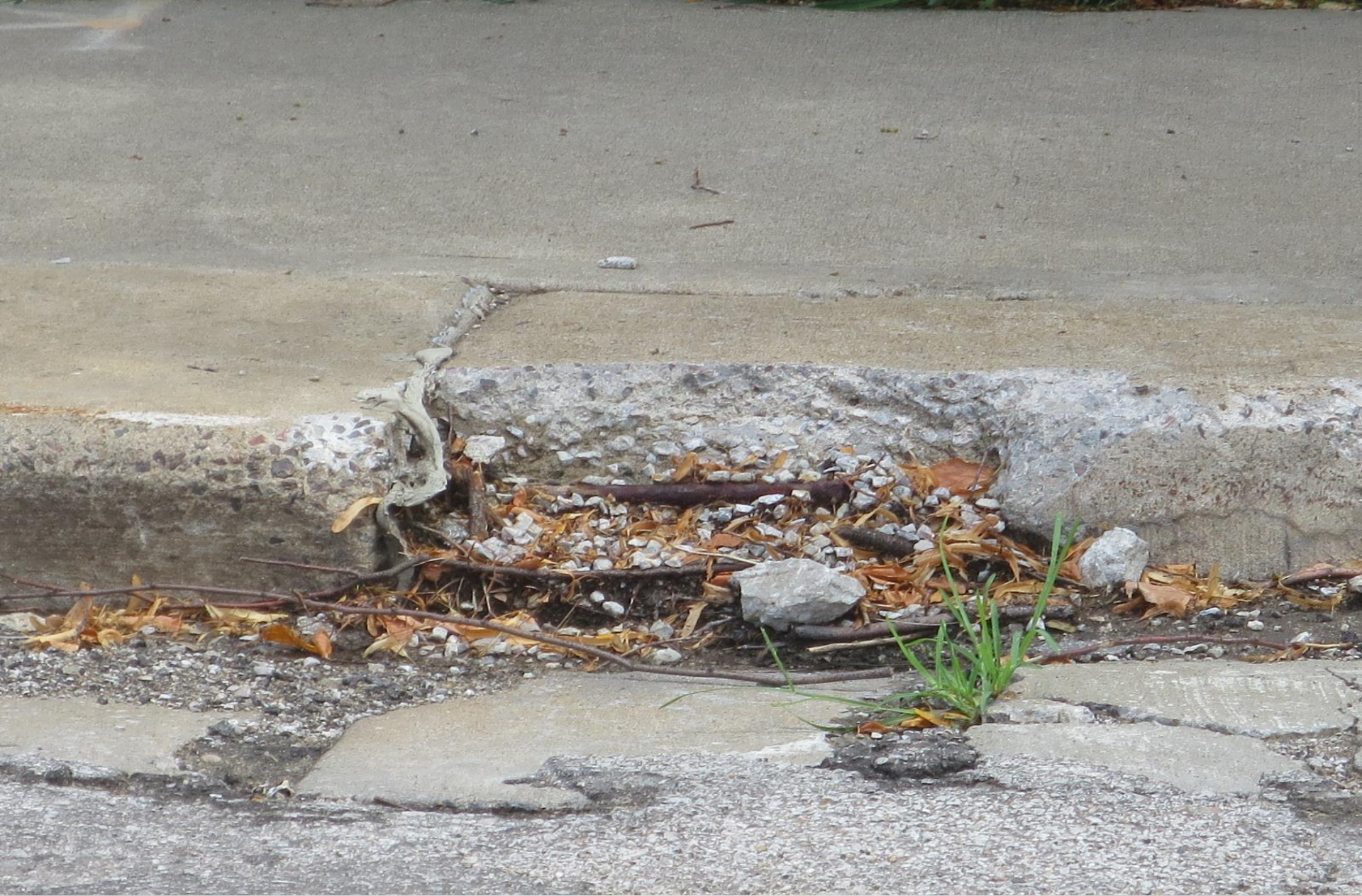
Damaged/Deteriorating Public Curbing On East Side Of Locust St. South Of Admiral Blvd.
