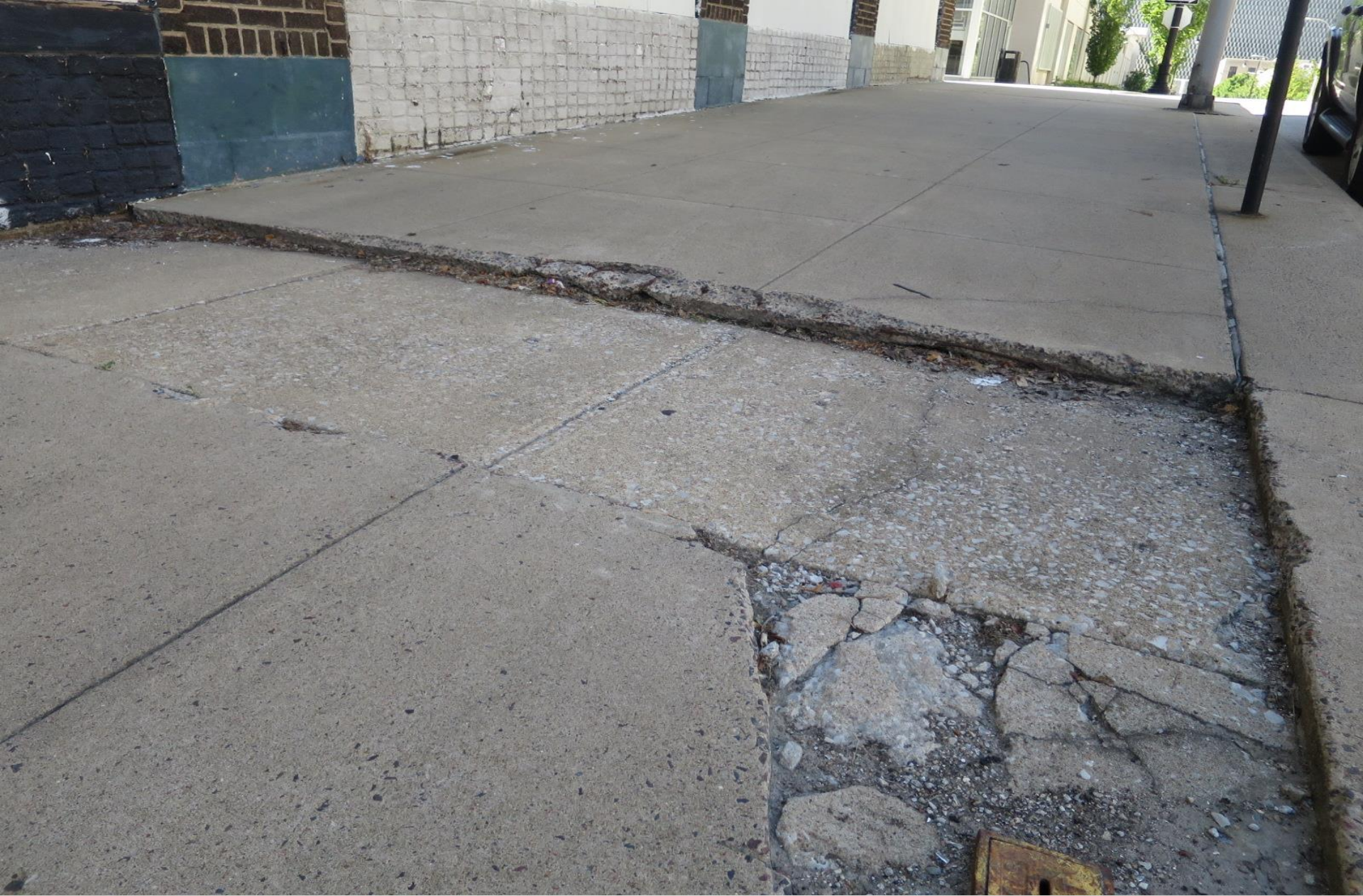
Trip Hazard In Deteriorated Public Sidewalk East Side Of Cherry St. South Of E 9 th St.
