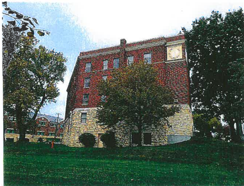
Photo 10: West elevation, view E, showing non-historic stair tower
