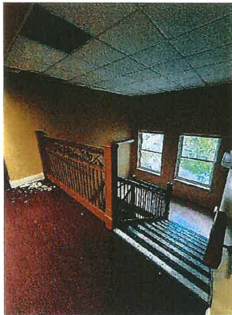
Photo 14: Fourth floor, detail of historic stair railing, view SW
