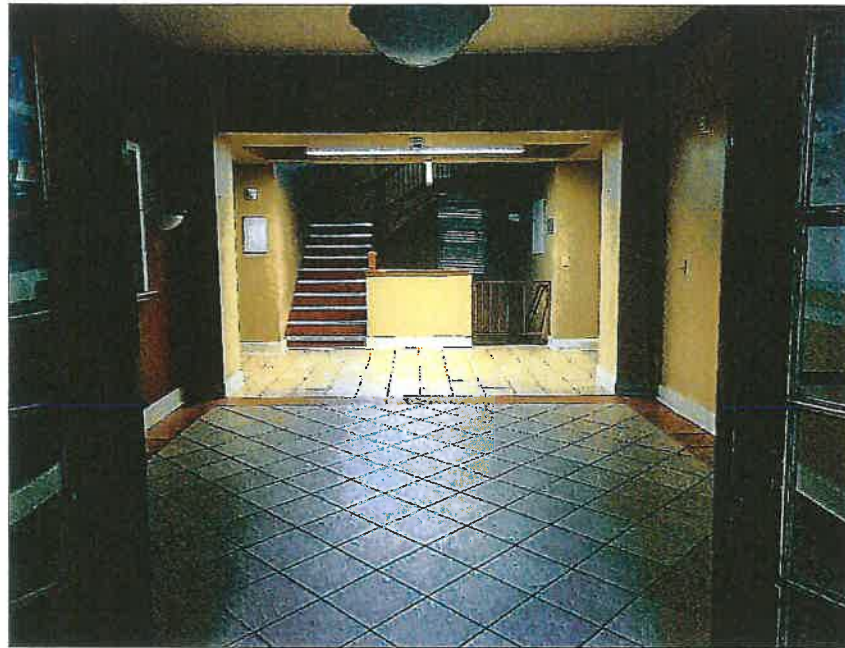
Photo 13: First floor, view NW from foyer, looking at historic stair
