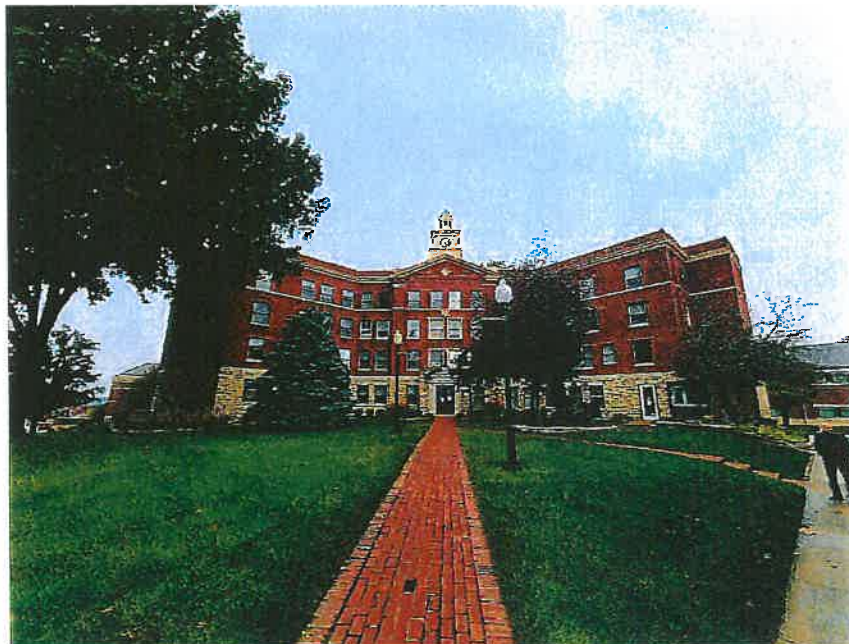
Photo 2: Façade, view NW
