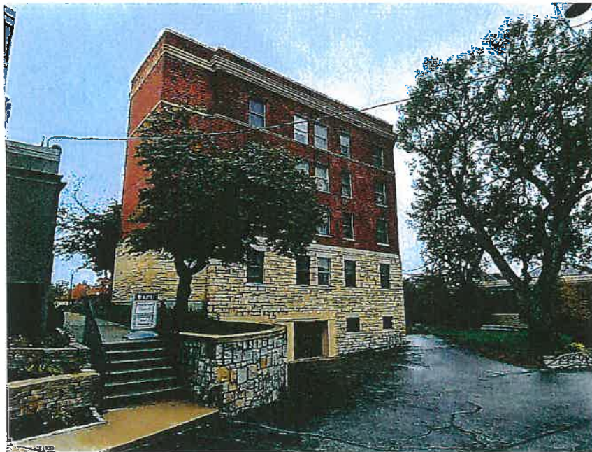
Photo 6: North elevation, showing historic retaining wall, view SW
