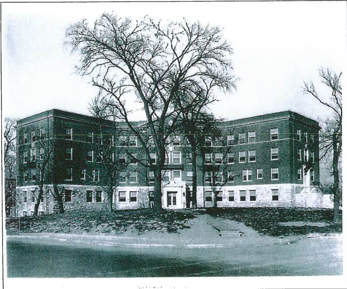
Figure 5: Undated photograph (pre-1940) of Smith Hall. Note the lack of cupola on roof and egress stair towers. Source: "Children's Mercy Nurses Home," General Collection (P1), Hospitals-Children's Mercy, Number 6, Missouri Valley Special Collections, Kansas City Public Library https://kchistory.org/image/childrens-mercy-nurses-home
