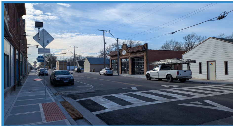
Figure 15. Roadway Improvements completed on Paseo in Downtown Marlborough
