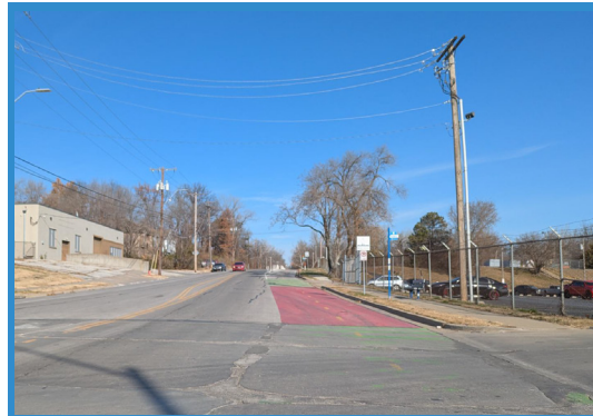
Figure 26. Roadway Conditions on Prospect Ave.
