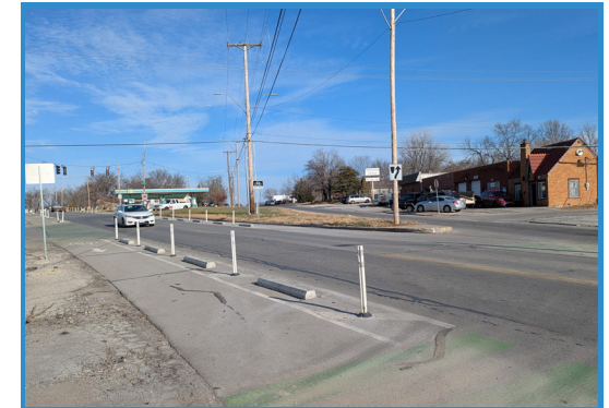
Figure 28. Infrastructure Condition on Hickman Mills Dr.
