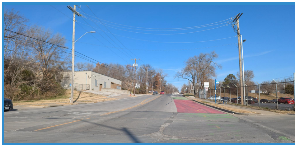
Figure 13. Roadway Section looking north at 85th St. and Prospect Ave.
