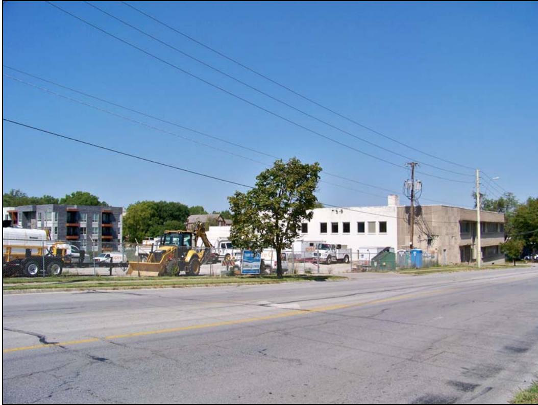
6500 Troost Ave – storage yard/parking lot, south elevation
