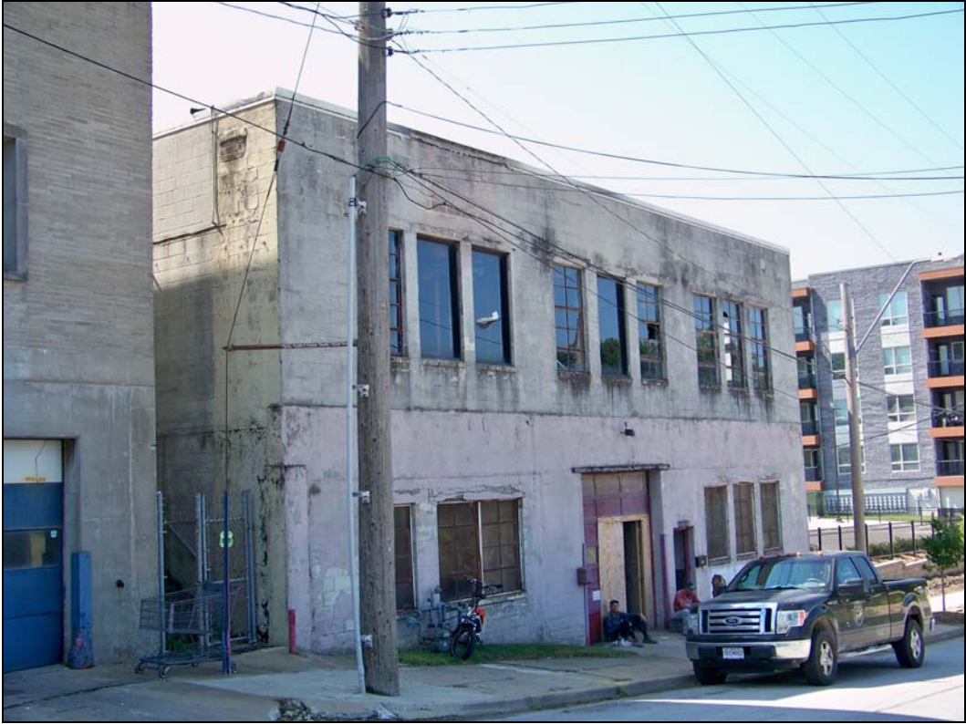
1015 E. 65 th Street – north elevation
