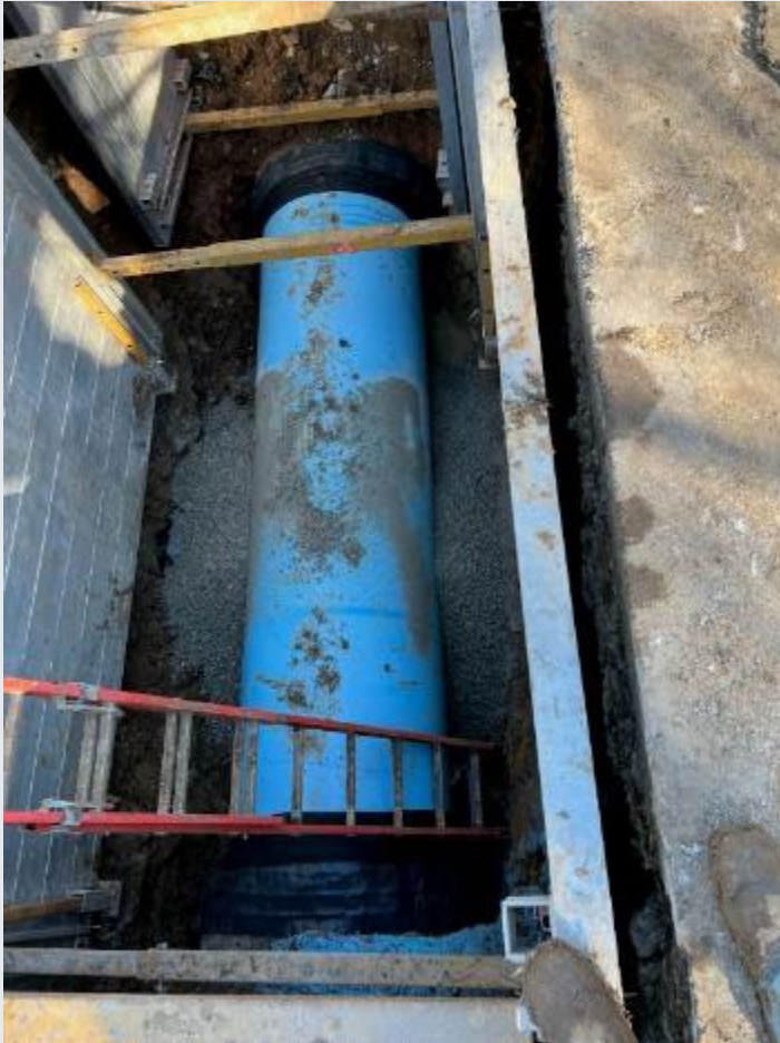
42-Inch Sewer Replacement
