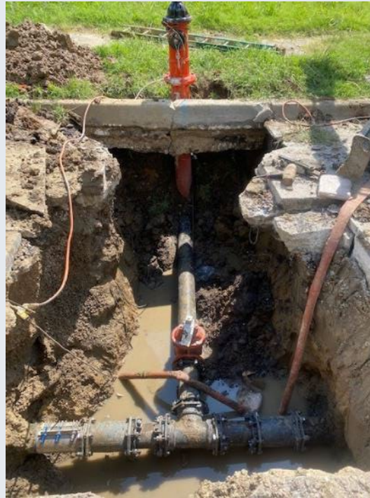
Examples of Fire Hydrant Repair Work
