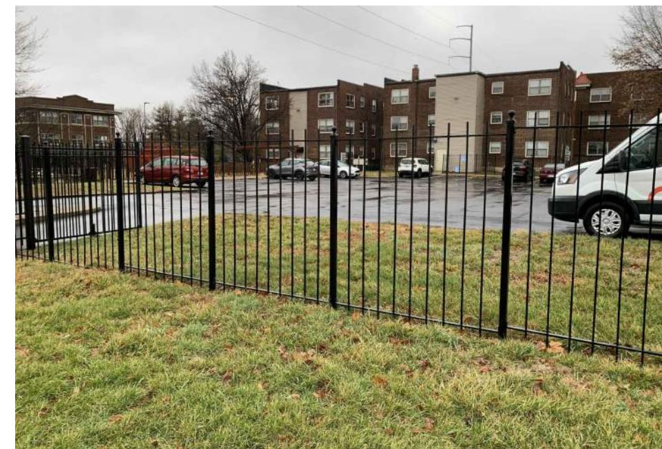
4' OR 6' TALL ANTI-CLIMB, ORNAMENTAL BLACK METAL FENCE EXAMPLE REF: PLAN FOR HEIGHT
