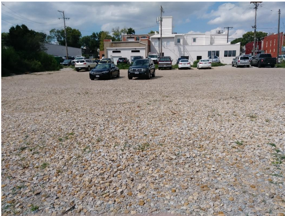
Gravel parking area does not conform to City standards for off-street parking; lack of stormwater control
