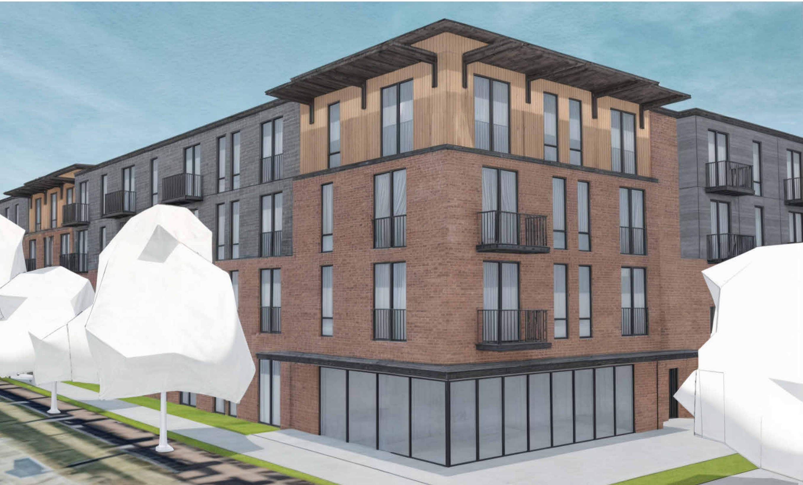
BUILDING 5 - CORNER OF 18TH & EUCLID
