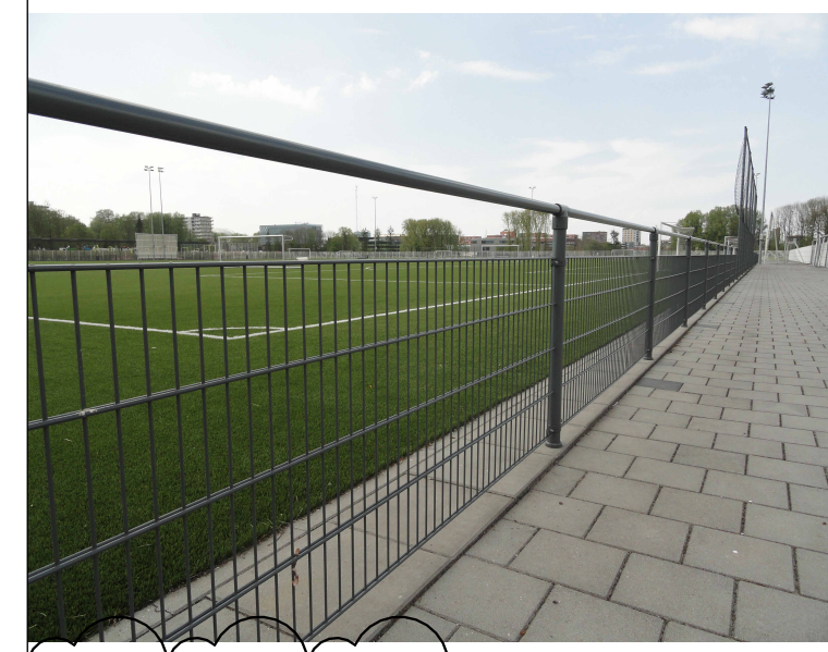
Proposed Fence Design Steel welded wire fence; painted black; transparency to be at least 80%
