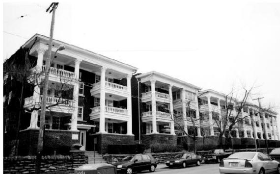
2. Combined Column Porch featuring columns that extend more than one story in height and support a smaller column of different material and design or the reverse — columns that extend one story and support columns that extend upward for several stories;
