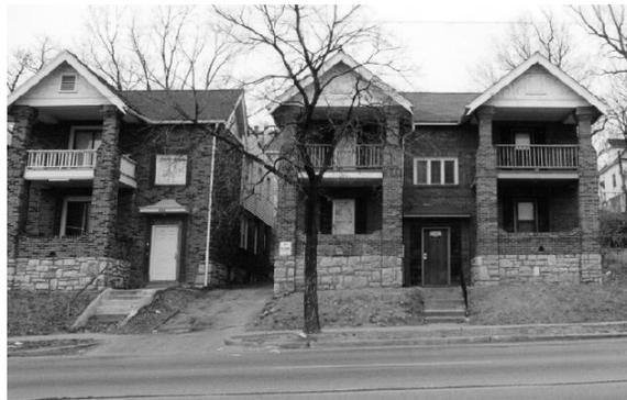
4. Transitional Enclosed Colonnade, this version retains the design of the original porch projections, but are enclosed and integrated with the interior living space.
